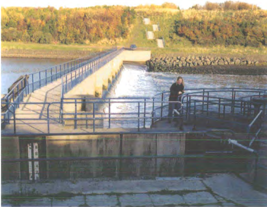
Figure 4-6 View of the Wansbeck barrage from the south-bank
