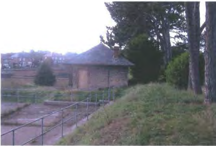
Fig. 109 Second valve house, within Filter Beds site, north side of Hexham Road, also listed grade 2 (7/31) and built in 1870 (copyright HER). The two valve houses are of completely different materials and design. This earlier house is stone built with ashlar quoins and a brick chimney. The later house above is brick built with ashlar dressings and decorative bargeboards and finials.
