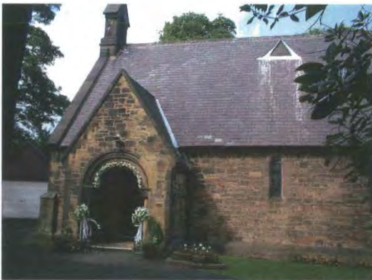
Fig. 55 Church of St. John, built 1866, designated as part of Local List (copyright author)
