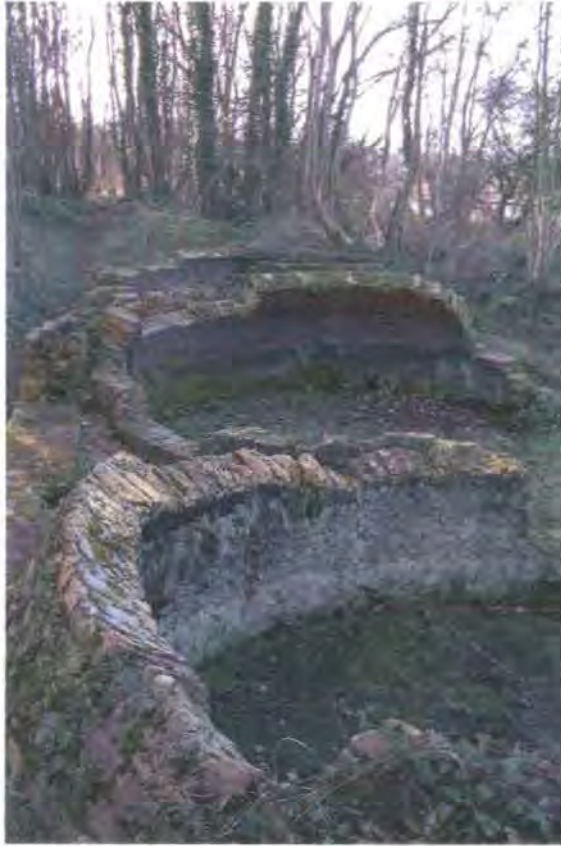
Fig. 91 Alongside coal, the Throckley Coal Company manufactured coke, mainly for use at Spencer's steelworks. A bank of twenty-two coke ovens was built using Stephenson's bricks, close to the Isabella Pit in 1869. They are shown on fig. 254. In 1875 the number of ovens was doubled and three years later a disintegrator for crushing the coal was added. In 1890 another twenty coke ovens were built. When new types of oven which could collect gases and by-products superseded the Beehive in the twentieth century, the complex went out of use (Ayrís and Linsley 1994). These fragmentary remains of four beehive coke ovens survive in the woodland at Newburn Country Park (copyright author).
