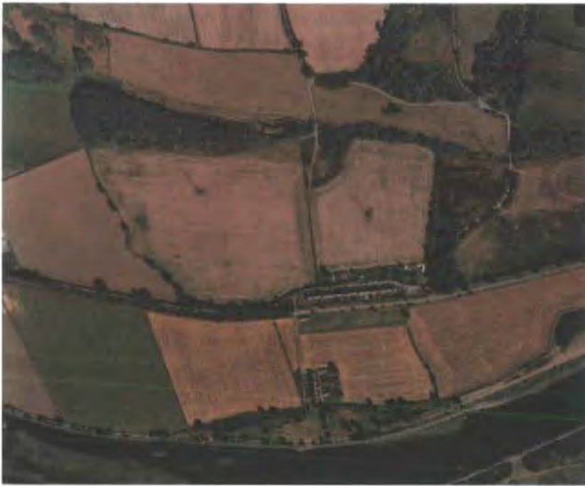
Fig. 96 Isabella Colliery reclaimed as Newburn Country Park (copyright R&I 14191084, 7 September 1991). The shape of the former coal workings is still apparent but the site is now grassed over and planted with trees. The west-east row of miners' cottages is Blayney Row and the north-south row is Moore Court (see chapter eight).
