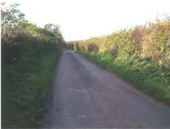
Fig. 140 Whorlton Lane looking west from Butterlaw Farm This sunken routeway was set out by 1767 (NRO Sant/Beq/9/1/1/24) following earlier field boundaries (copyright author).
