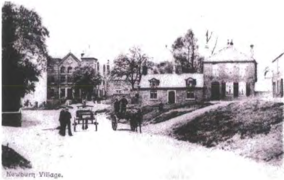
Fig. 26 Postcard of Newburn High Street c. 1900 (copyright NCL acc. 70719). The grand towered building on the left which still stands is the institute built by Thomas Spencer; that on the right, which has been demolished, is Newburn dairy.
