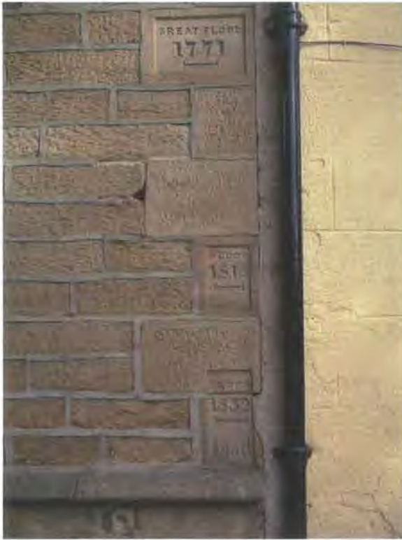
Fig. 126 The heights of former floods at Newburn, shown on the wall of the Boathouse Inn. (copyright author)
