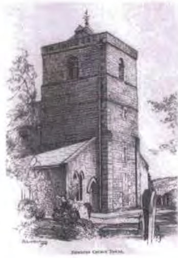
Fig. 170 This drawing of Newburn Church by Robert Bartram, 1928 (after Dodds 1930) shows the oldest part of Newburn church, the early Norman tower which incorporates Roman stones from Hadrian's Wall. The tower is in three stages. The first has round-headed windows and a blocked west door, the second has slit openings and the third stage has round-headed belfry openings. The tower has a pyramidal roof and weathervane (listed building 7/26).
