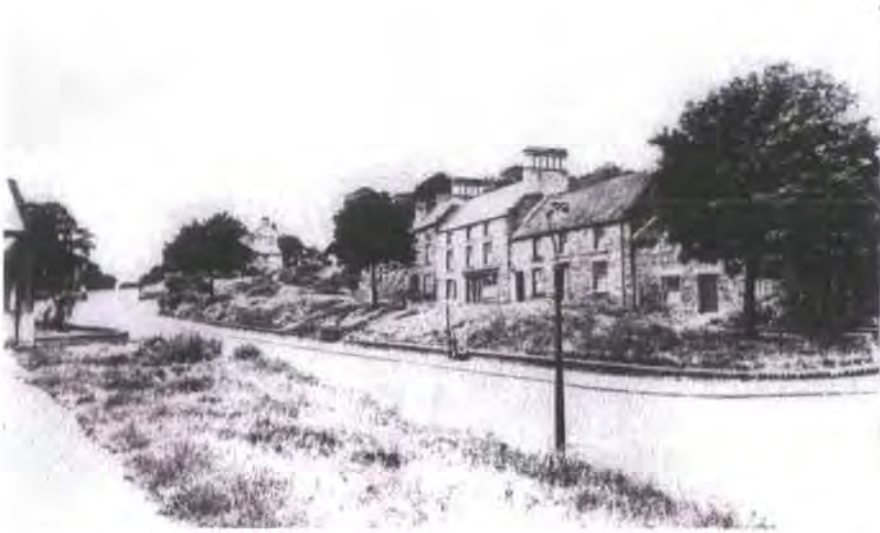
Fig. 20 Front Street became Newburn High Street and was built over the village green by the mid nineteenth century (copyright NCL acc. 57655). The houses shown here no longer exist.
