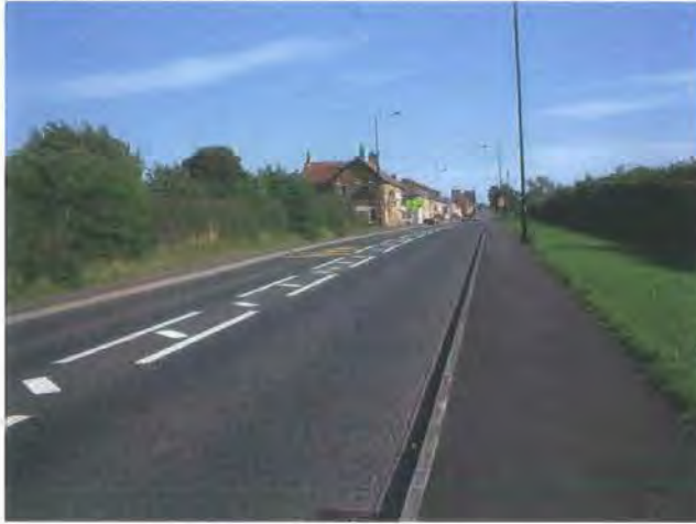
Fig. 137 General Wade's Military Road, the Newcastle to Carlisle toll road, built 1752-3, now Hexham Road, looking east towards the former Engine Inn and Hawthorn Terrace, Walbottle. (copyright author)
