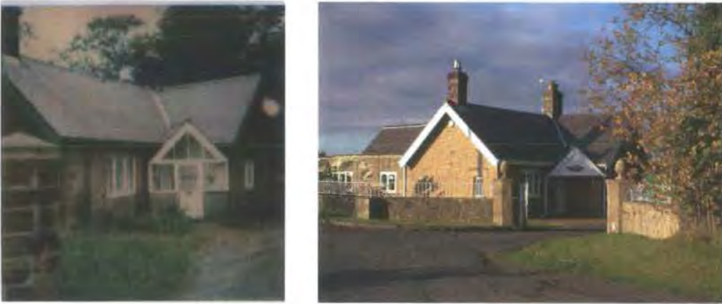
Fig. 54 Lodge to Whorlton Hall in 1980s (copyright HER) and 2006 (copyright author). The gate lodge was added to the parkland by 1898.
