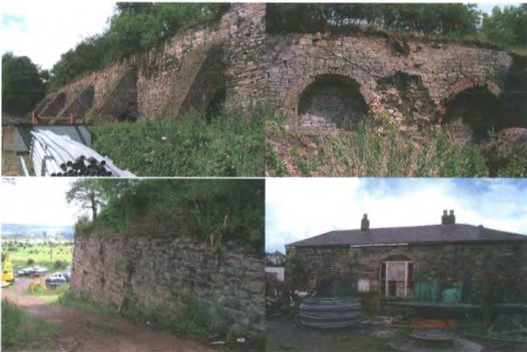
Fig. 115 Remains of Tyne Iron Works – a number of large stone buildings and retaining walls survive. The prominent arches in the top right photograph may have housed puddling or re-heat furnaces or may simply represent a viaduct ramp to the blast furnace top (HER 4346). Another prominent ramp seems to incorporate rooms. In a long stretch of rubble-built wall, the former doorways to the workers' houses can be seen (Grundy et al. 1992, 374). The bottom right photo is the grade two listed (10/25) manager's house of c. 1830 (copyright author).
