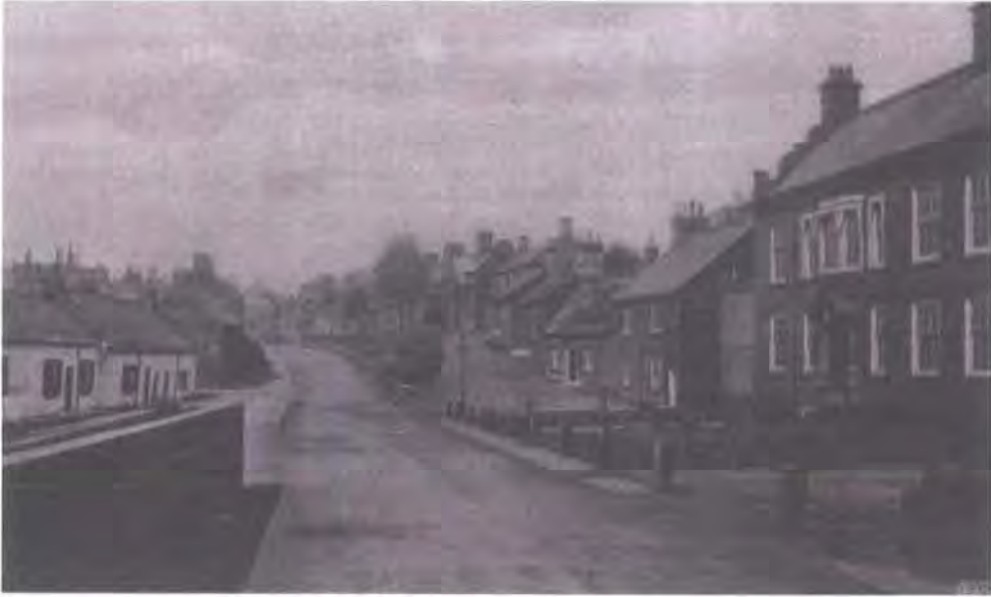
Fig. 28 Further east along Newburn High Street, c. 1913 (copyright NCL acc. 51492). Spencer's Steelworks office is the grand building on the right foreground which still exists. The single-storey whitewashed cottages on the left have now gone, as have the cottages on the right in-between Spencer's office and the Duke's House. The buildings are discussed in chapter eight.
