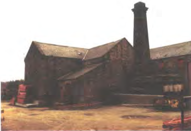
Fig. 69 Whorlton Grange – the presence of the chimney shows that this was a mechanised farm, with an engine powering the threshing machine (copyright HER). Farm mechanisation was a key feature of the 'High Farming' era of the nineteenth century.
