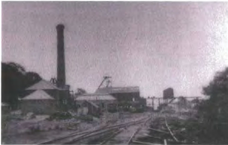
Fig. 90 Isabella Colliery, owned by Throckley Coal Company, was in operation from 1869 to 1954 (copyright L. Walton, after Walton 1994). This photograph shows the infrastructure associated with the mine including the mineral railway and coal drops.
