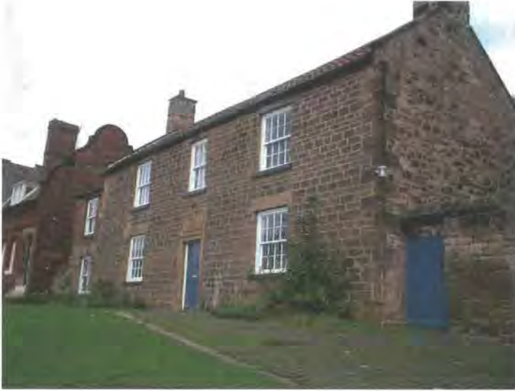
Fig. 183 Duke's House, High Street, Newburn (copyright author) This attractive property is built in coursed squared sandstone and has a raised crescent (the Duke of Northumberland family emblem) over the front door (listed building 7/35).
