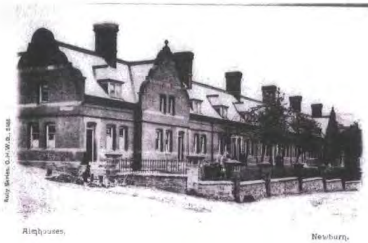
Fig. 185 Postcard of Newburn almshouses (copyright NCL acc 70723). The design of this building is interesting. The shaped gables echo the Dutch gables common in the seventeenth century (for example Holy Jesus Hospital and King Charles House, Newcastle). The design was copied in Spencer's Steelworks office building (figs. 121-123).
