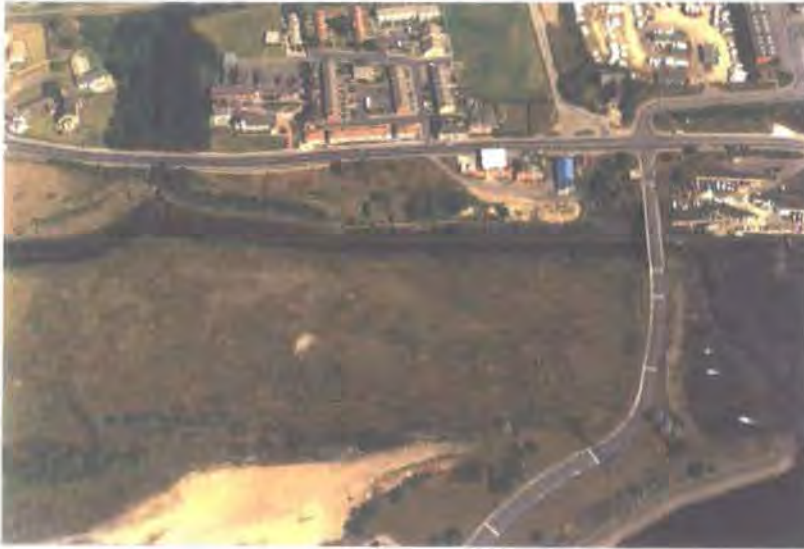
Fig. 30 Lemington Gut - the original course of the River Tyne became a dammed canal-like narrow water course after river improvement work in 1876 (copyright Air Fotos, n.d.). The impact of this work is discussed in chapter six.
