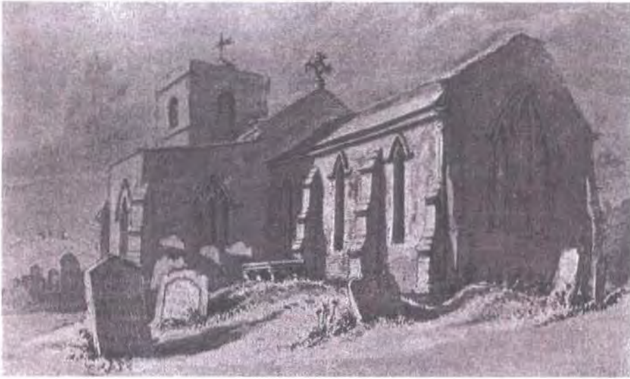
Fig. 172 Painting of Newburn church c. 1840 (after Dodds 1930, 127). In 1827 alterations, including the installation of new mullions at the windows, were carried out. The windows on this painting and the sketch above are very different. These gothic style lancet windows are typical of the nineteenth century Early English style (Wild 2004, 73).
