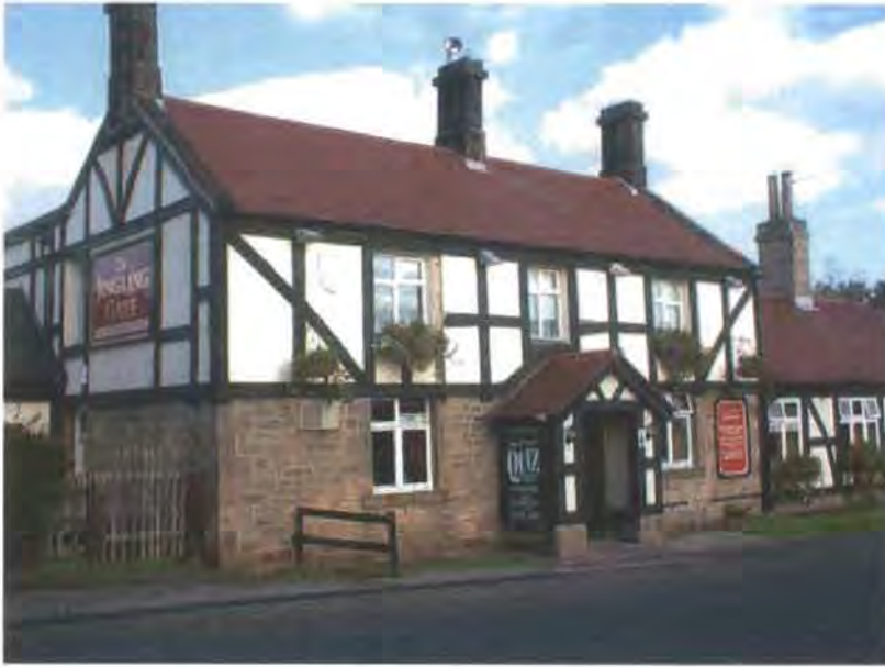
Fig. 53 Jingling Gate Public House, Stamfordham Road 2006 (copyright author). The fine building shown on the photograph above is hidden under a mock 'Tudorbethan' façade, a porch has been added, a door and the gable-end window blocked up and the remaining sash windows have been replaced by plastic frames.
