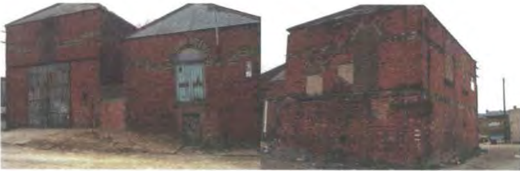
Fig. 85 Disused colliery buildings built by the Throckley Coal Company at Blucher Pit (copyright HER, circa 1994). These buildings have since been demolished. The buildings comprised of the former winding engine house, boiler house, workshops and pithead baths. One building displayed a date stone of 1900. Of some architectural merit, this complex was not deemed worthy of listing by the Monument Protection Programme Assessment, due to being of low technological importance and poor examples of their type.
