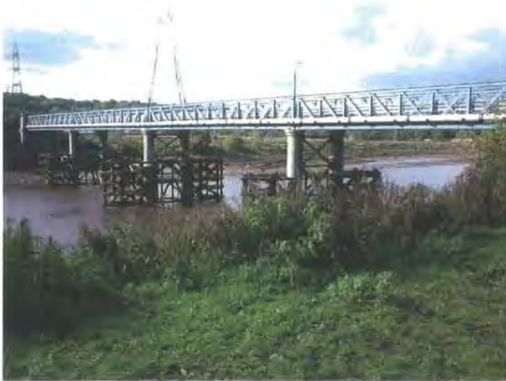
Fig. 130 Newburn Bridge, included on Newcastle City Council's Local List, provided a river crossing once the ford had been dredged away in 1876 (copyright author).
