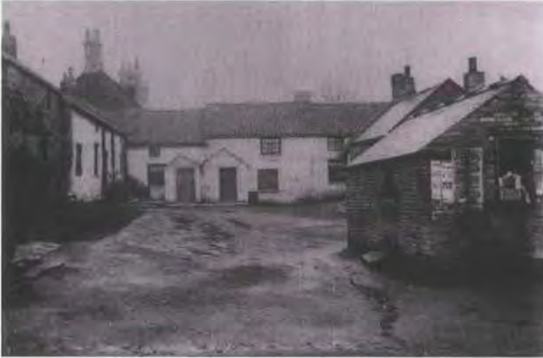
Fig. 50 These cottages at High Square, Walbottle c. 1900 were amongst the earliest casualties of change, demolished in the 1930s as part of an extensive 'slum clearance' by the council (Twas UD/Nb/40/33; copyright NCL plate 5431 neg. 8/11/83 & 25/8/84 acc. 36501).
