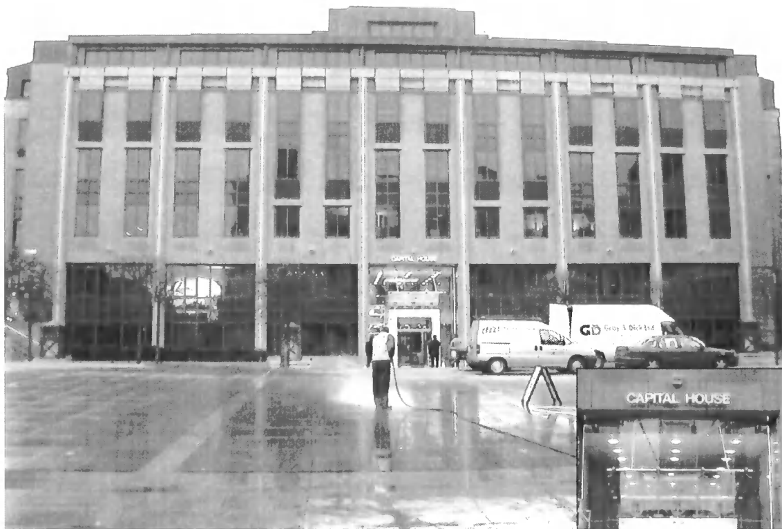
Figure I.13: Capital House and its entrance with slab cleaning in progress.
