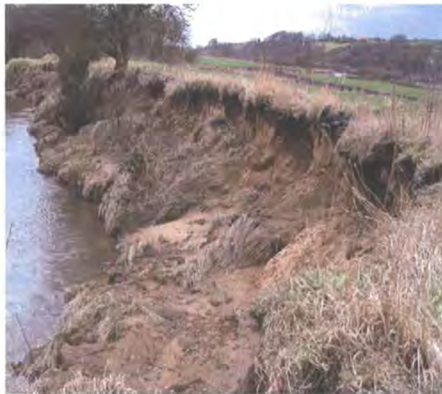
Figure 6.12: Extensive channel bank slumping of the main Esk (near Duck Bridge)
