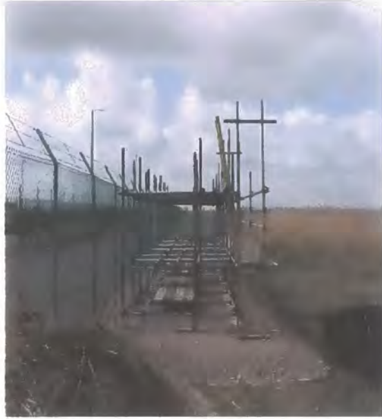
Plate 2.2. The scaffolding structure before the test beds were put in place
