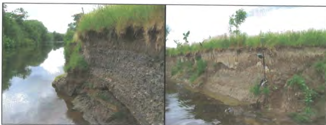
Figure 4.15: Comparison of river bank composition between High and Low Stock Bridges: a composite bank with a thick non-cohesive layer (left), and an almost completely cohesive bank (right).
