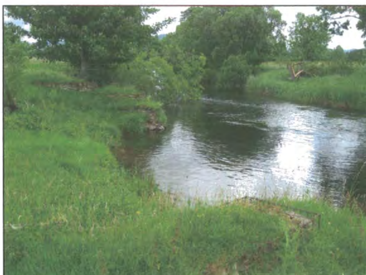
Figure 4.44: Gabion cages between Portinscale and High Stock Bridge (NY 247 251, looking upstream).
