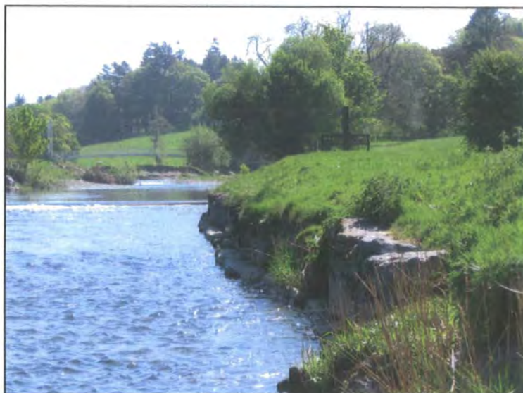
Figure 4.43: Boulder revetment wall at Portinscale (NY 251 238, looking upstream).
