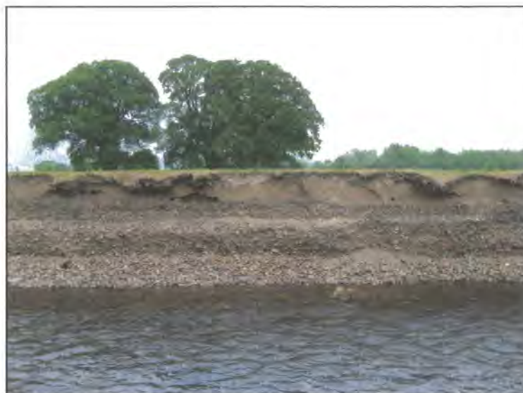
Figure 2.14: A well-developed, eroding composite river bank near Portinscale Bridge (height c. 2.5 m). Note the cohesive upper layer of fine-grained sandy material overlaying a non-cohesive lower layer of coarse pebbles and gravel. The turf slippage and slight overhang development at the bank top, and the steepened profile of the lower bank suggest recent active erosion of this bank.
