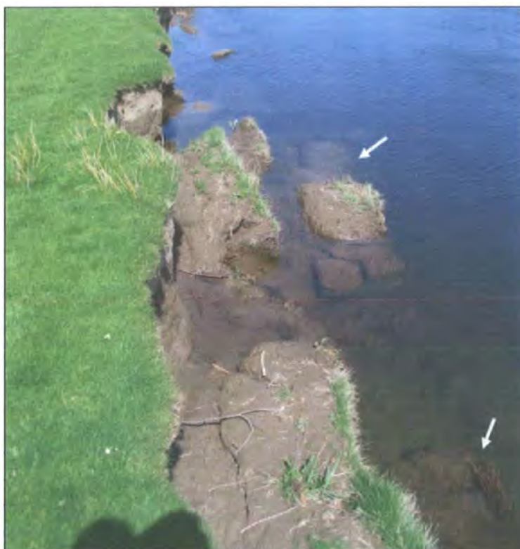
Figure 4.28: Unvegetated, intact blocks (indicated by white arrows) lying in the river channel below more recent failures at bank 6 (flow direction: away from photograph).
