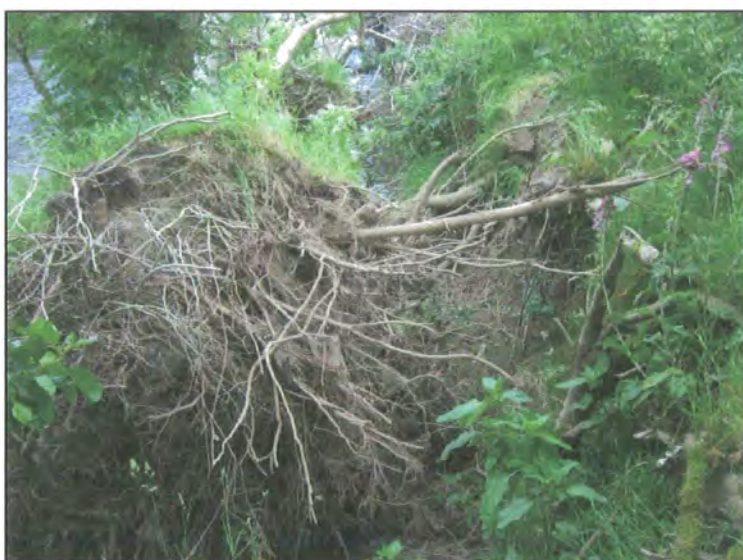
Figure 4.31: Collapsed bank-top tree at NY 247 251, showing a considerable amount of material removed from the bank attached to the roots, and a steep bank face left exposed by the removal of the material.
