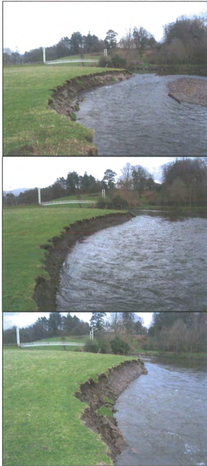
Figure 4.23: Block failure events and material removal from bank 3 near Portinscale suspension footbridge (looking upstream). Photograph dates: Top - 19 th February 2007, middle – 5 th March 2007, bottom – 11 th March 2007.
