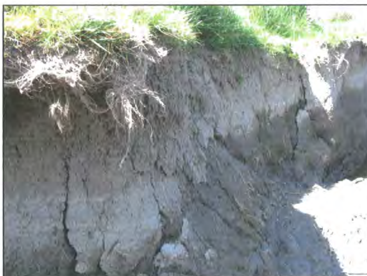
Figure 2.19: A desiccated river bank on the River Derwent near Bassenthwaite Lake, showing a dry and crumbly upper bank with deep cracks in the upper bank surface.
