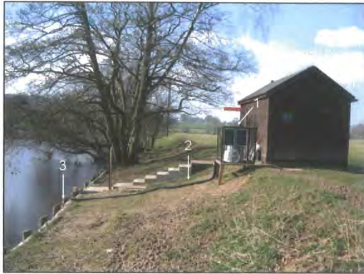
Figure 3.4: Field monitoring station at Ouse Bridge. The elevated cage (1) contains the automatic water sampler and datalogger (not visible). The black pipe (2) leading down the bank contains the turbidity probe wire, water sampler tube, sampler float switch and pressure transducer. The turbidity probe and water sampler tube are attached to the bank face at the stilling well (3). The two solar panels on the cage supply power to the datalogger battery. The hut close to the cage is an Environment Agency river level and flow gauging site, which collects river stage and discharge data.
