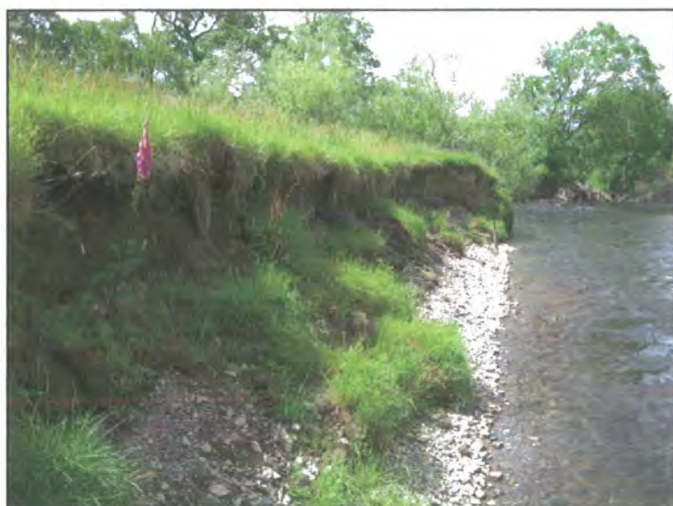
Figure 4.25: Bank 5 (West bank, NY 243 259, looking downstream).
