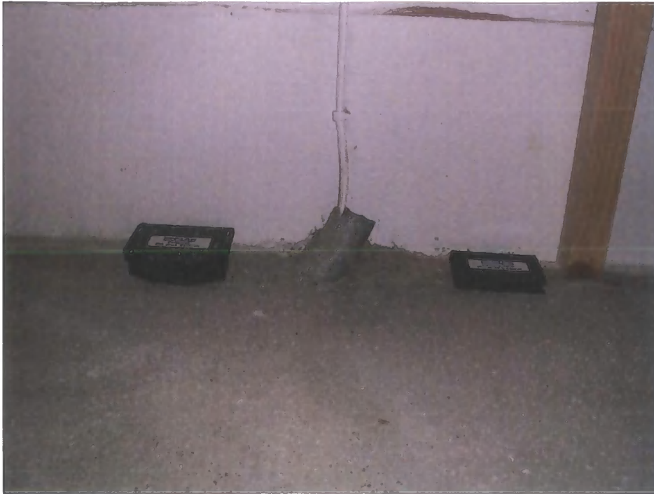
Figure Twenty-Nine. The placing of baits stations along floor-wall joins, performing the lines of neophobic rat movement. Source: Own photo.
