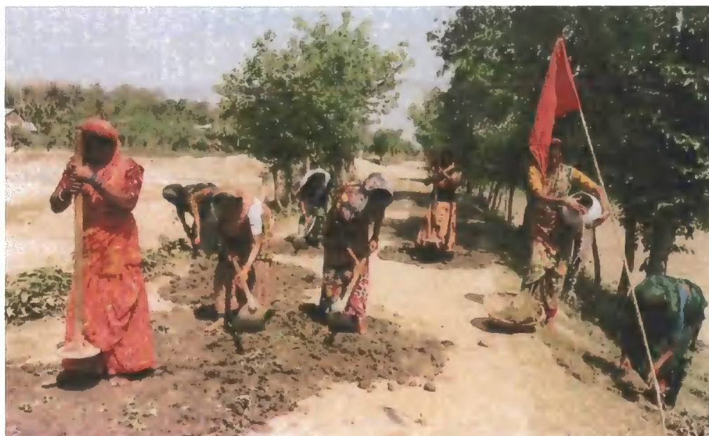
Figure 5.2: The RMA women are maintaining the rural earthen roads to keep it passable year-round (Photo: RMP/CARE)
