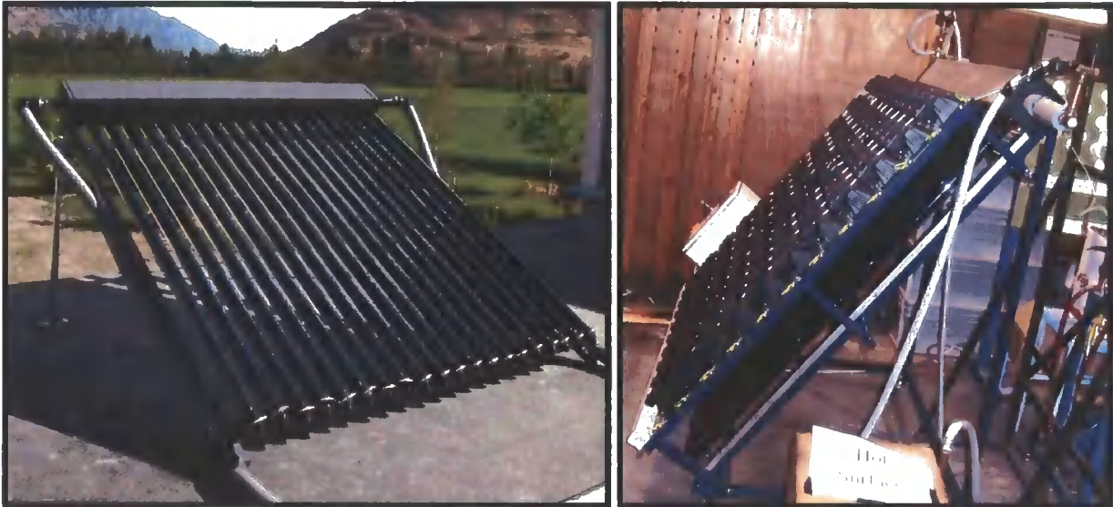
Figure 8-1: Evacuated tube solar collector panel and light flux
