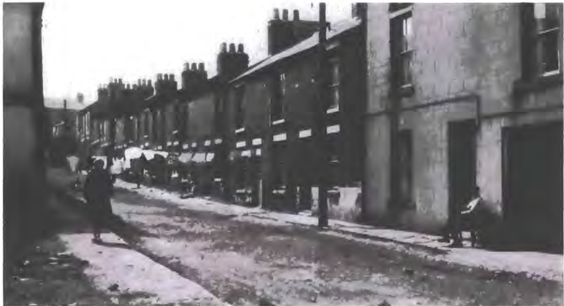
Plate 3.1: Category D Settlement (Townsend and Couper, 1970; courtesy of Durham County Council).
