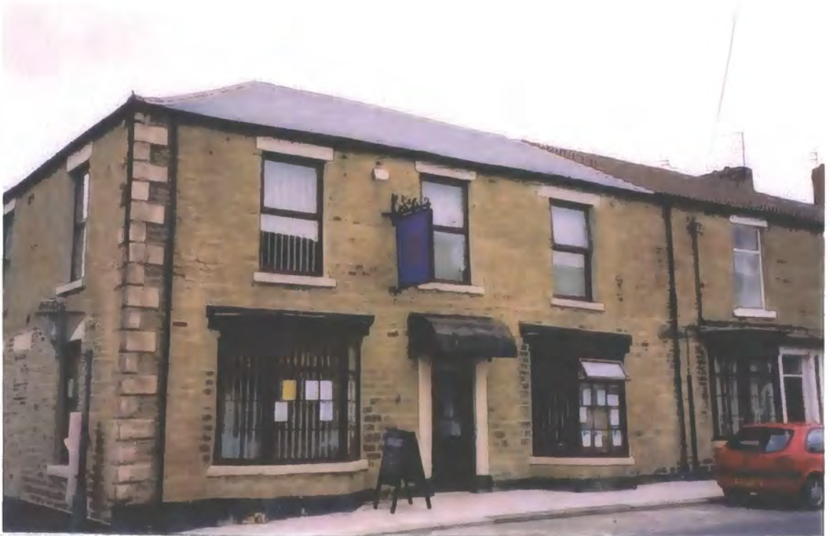
Plate 4.10: Dene Valley One Stop Shop operational.
