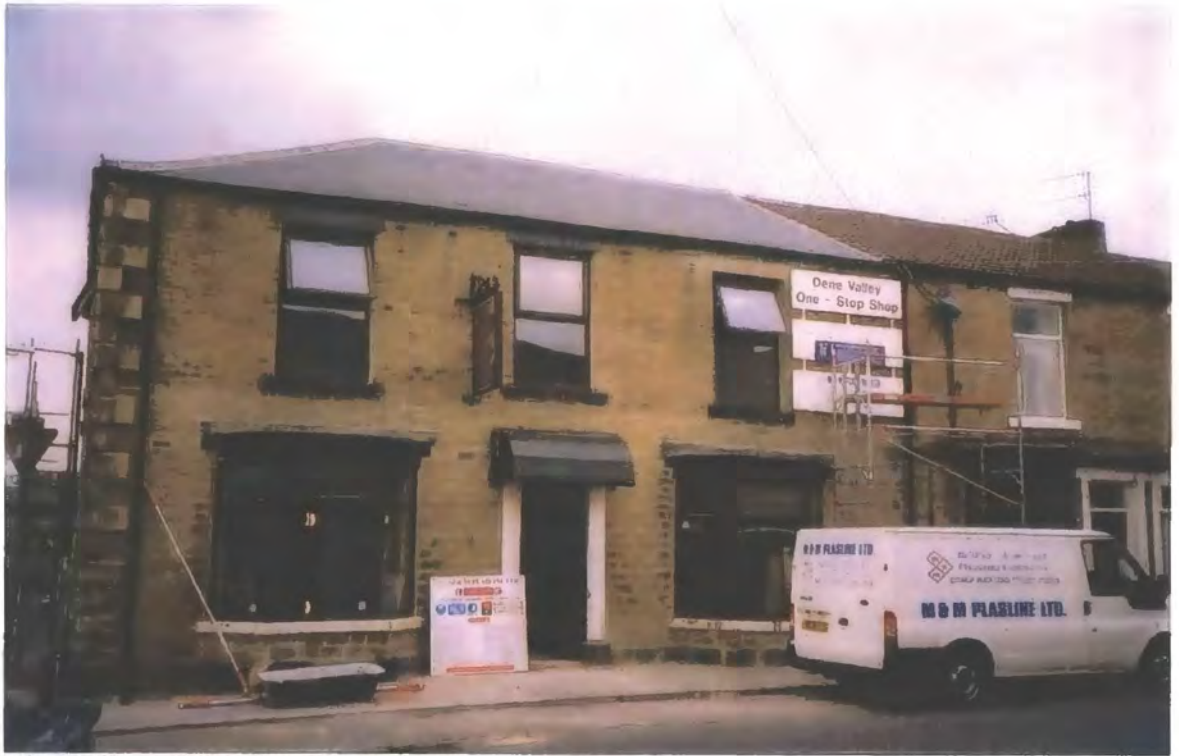
Plate 4.9 Dene Valley One Stop Shop under construction.
