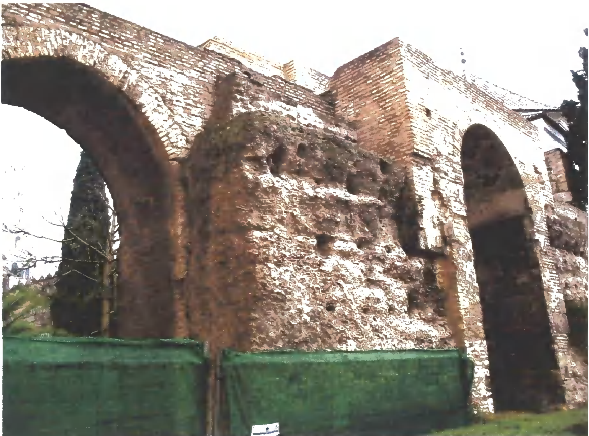
Figure C.82 Se1 Seville Alcazar rammed earth wall
