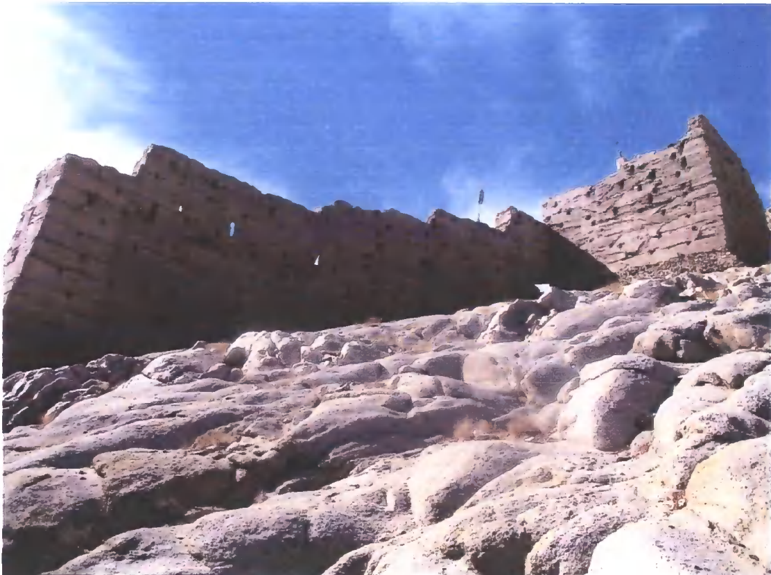
Figure D.23 Sh1a Shey Palace rammed earth wall north side photograph
