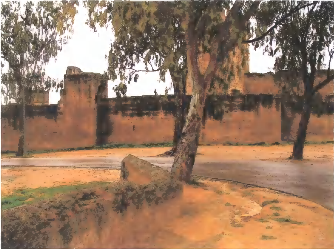
Figure C.7 Al3a Curtain walls constructed 1471
