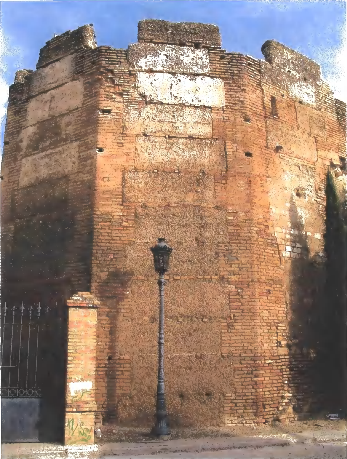
Figure C.79 Pa4 Octagonal and brick tower
