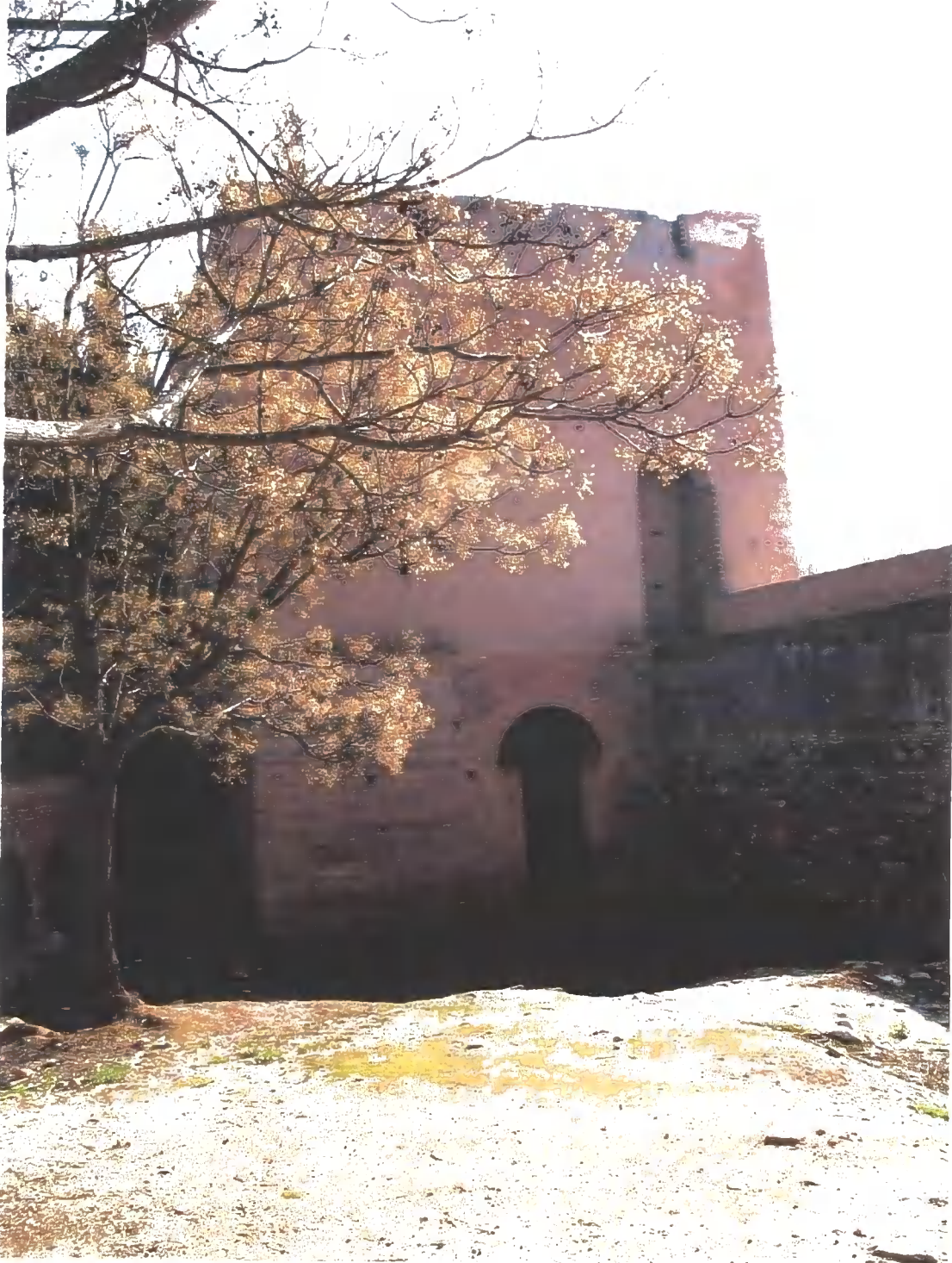
Figure C.53 Gr6 Water tower ( Torre Agua )
