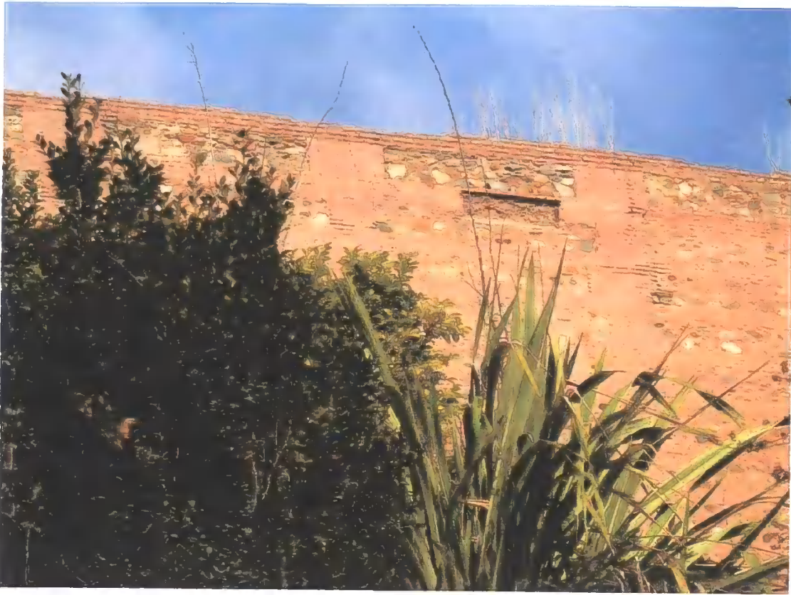
Figure C.51 Gr4b Nasrid wall repaired
