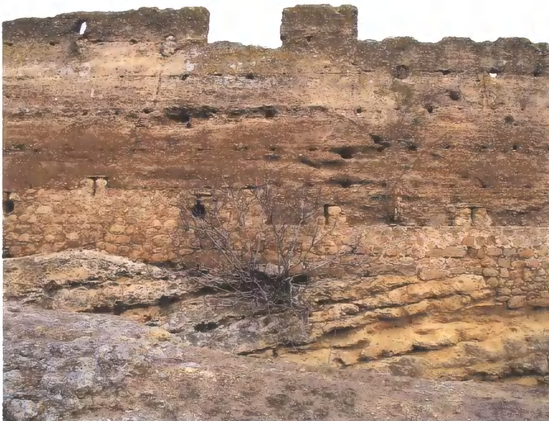
Figure C.27 Ca3 Exterior wall. Rock foundation with masonry levelling course.
