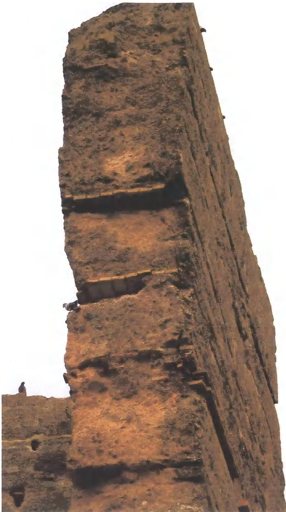
Figure C.25 Ca1b Bricks over putlog hole
