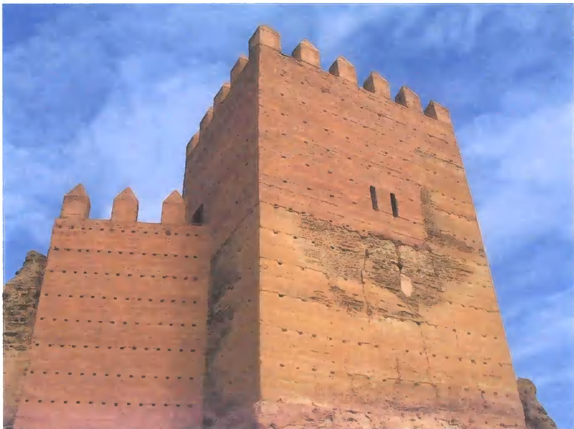
Figure C.87 Ta4 Tabernas repaired face
