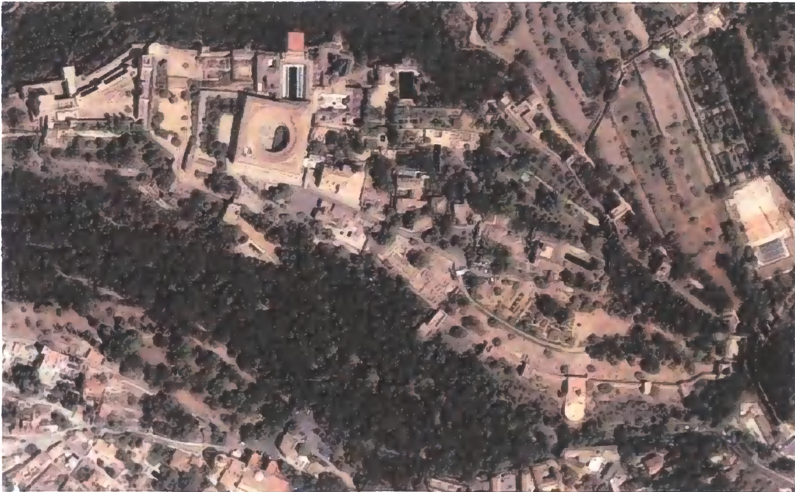
Figure C.45 Aerial photograph of the Alhambra
