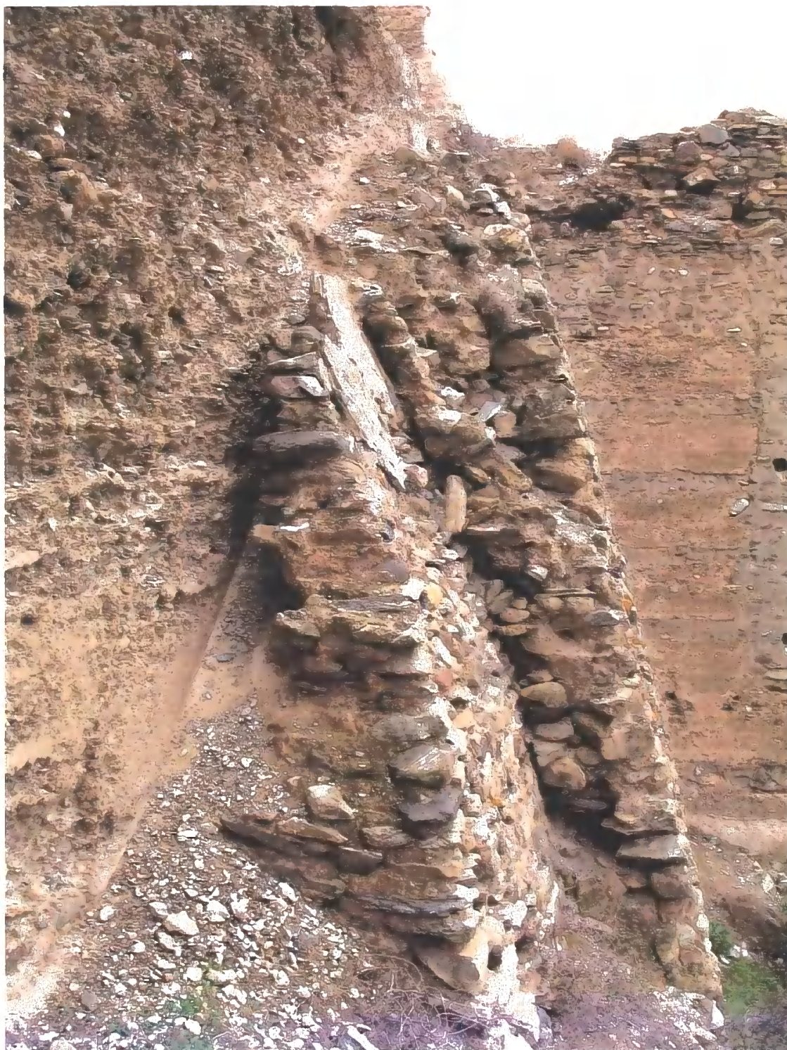
Figure C.88 Ta1 Rubble facing to rammed earth
