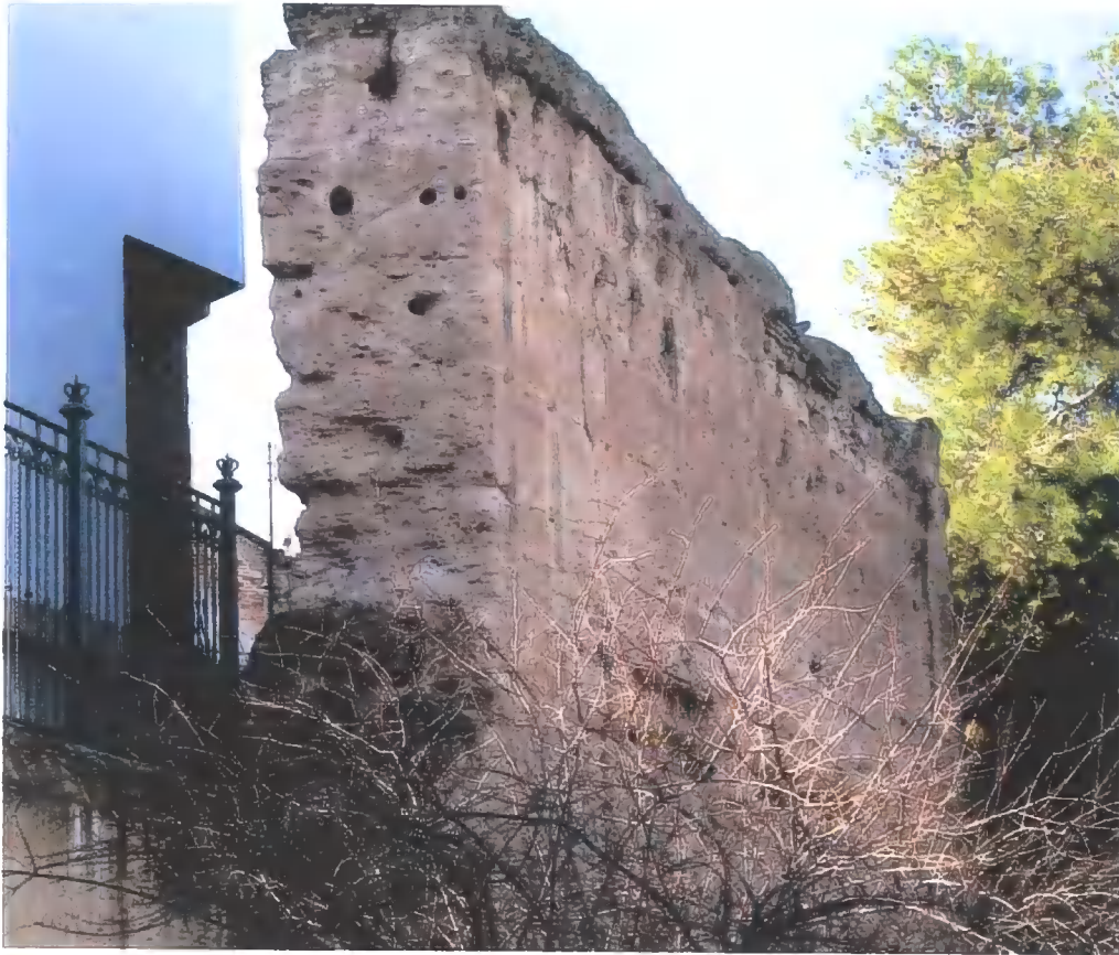
Figure C.63 Ra2a Section of La Rambla town wall
