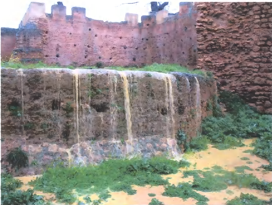
Figure C.8 Al3b Retaining section of curtain wall, probably constructed 1471
