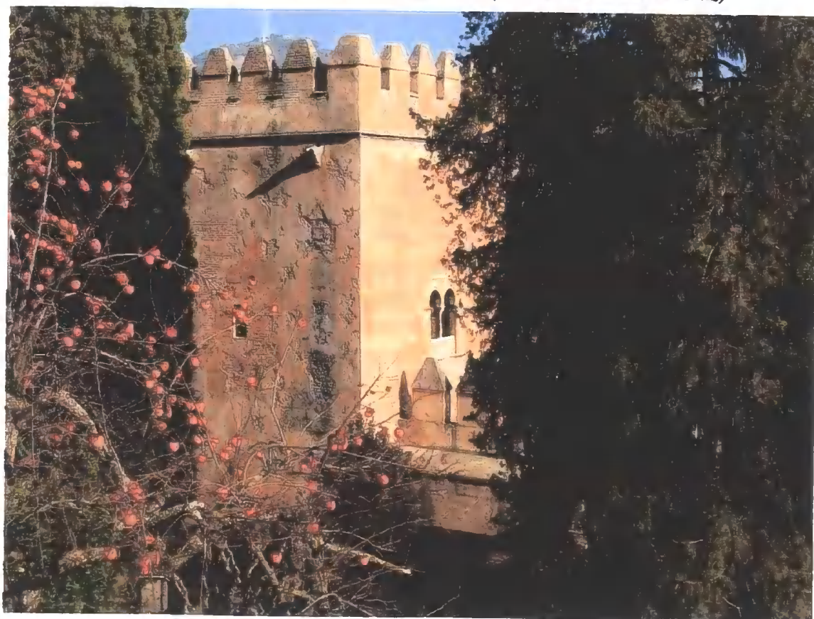
Figure C.55 Gr8 The Spiked tower. Spikes visible below crenellations, casting long shadow.
