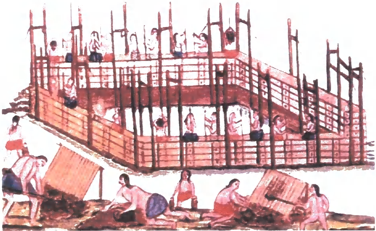
Figure A.8 Rammed earth formwork South America
