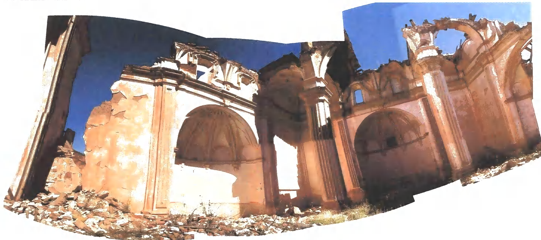
Figure B.35 Vi2 Villafeliche chapel internal, looking north east
