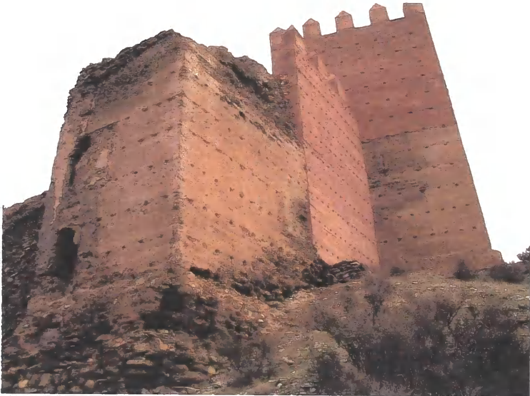
Figure C.89 Ta4b Tabernas repaired face
