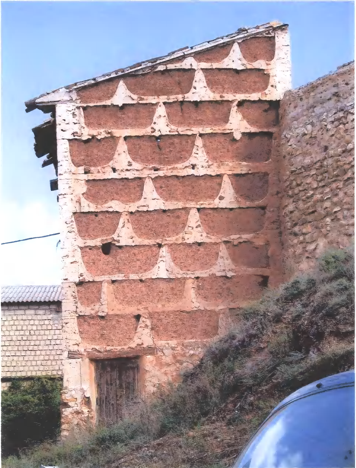
Figure B.30 Vi1 Villafeliche barn gable end photograph
