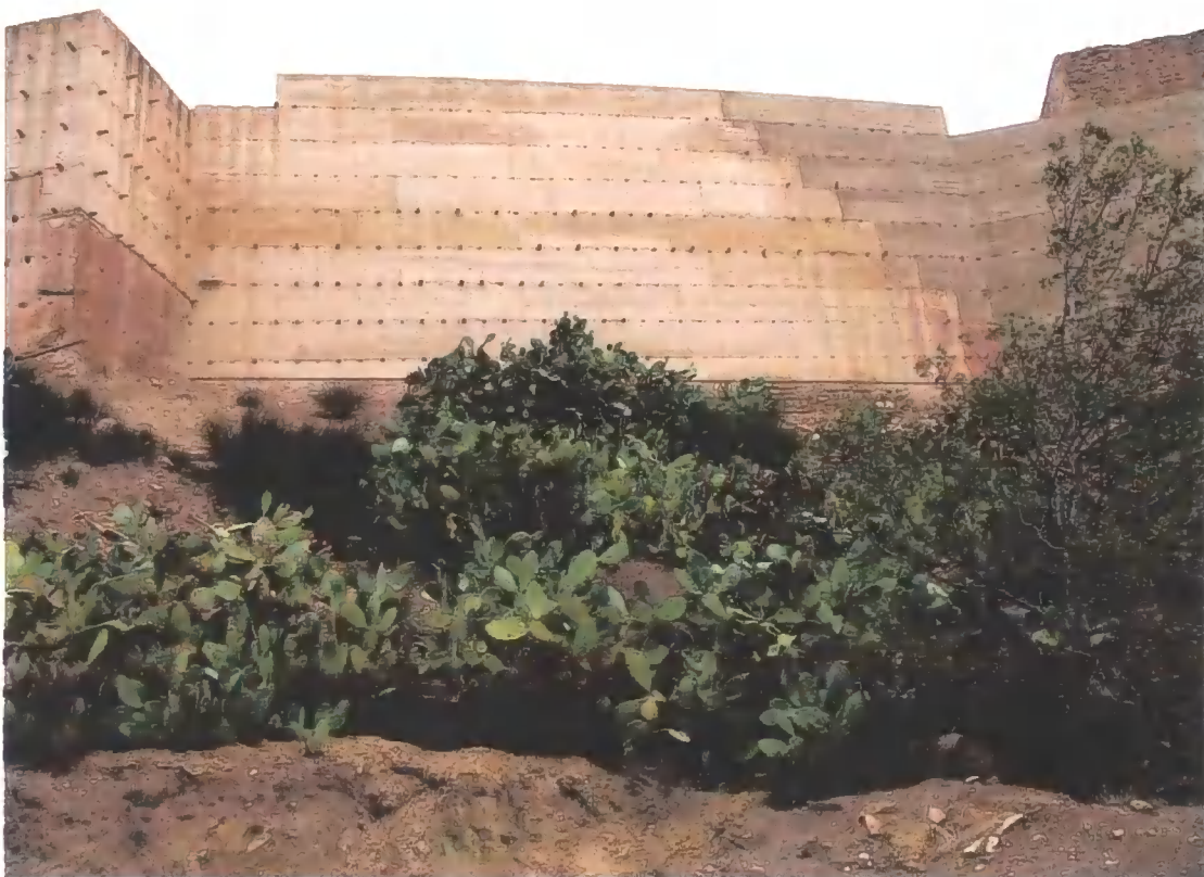
Figure C.74 No4 Concrete repair to south face of curtain wall
