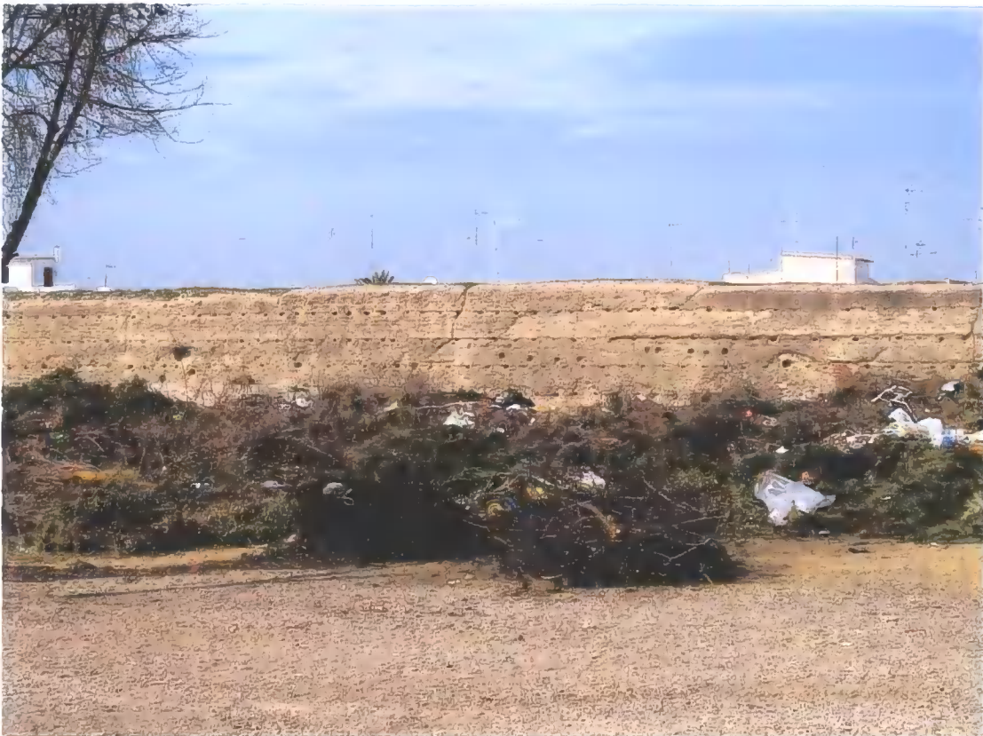
Figure C.76 Pa1 Muslim castle internal. Now used as town garbage wagon park
