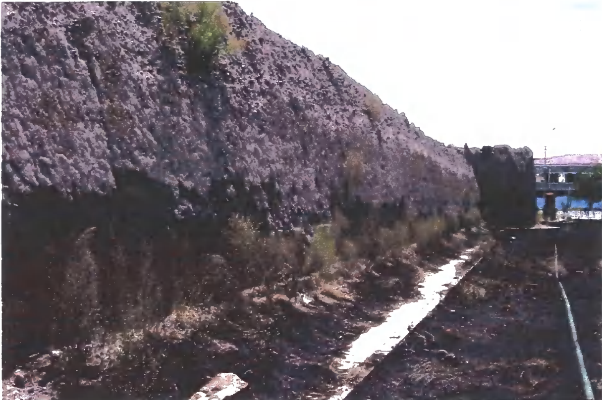
Figure A.7 Rammed earth wall at Yerevan, Armenia (Hurd 2006b)
