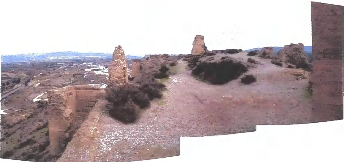
Figure C.90 Ta5 Tabernas internal view
