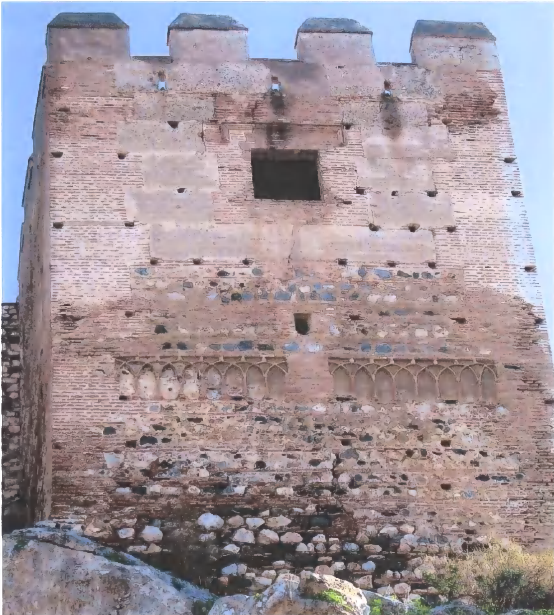
Figure C.81 Sa1 Salobreña castle, constructed before 1408
