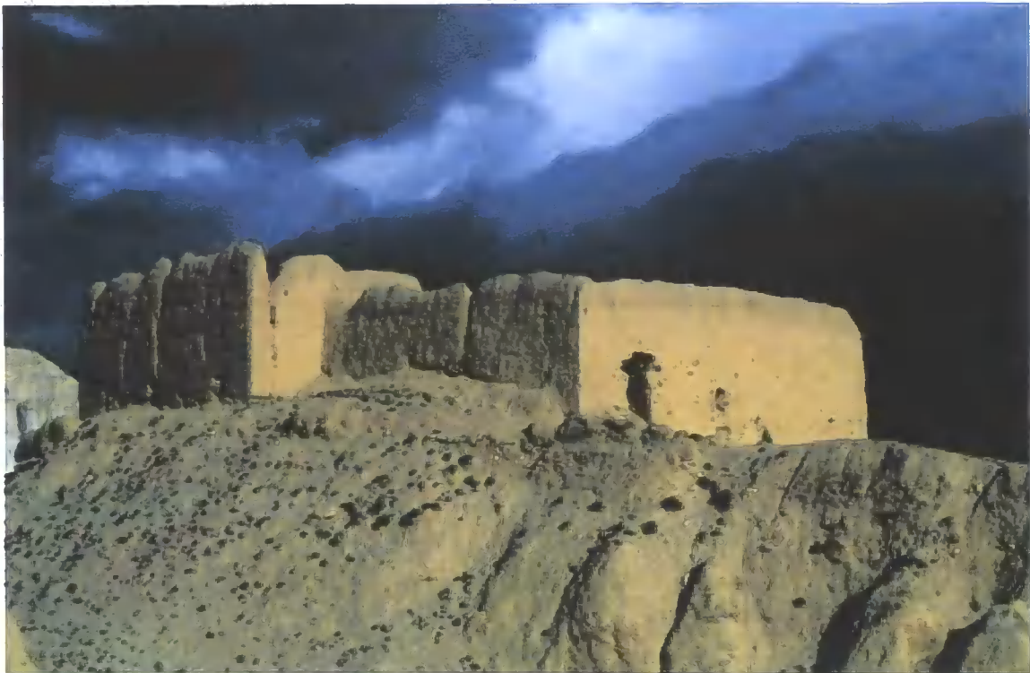
Figure A.5 Rammed earth in Mustang, Nepal
