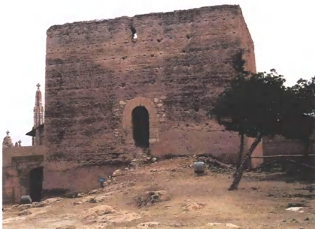
Figure C.72 No2 12 th century rammed earth tower
