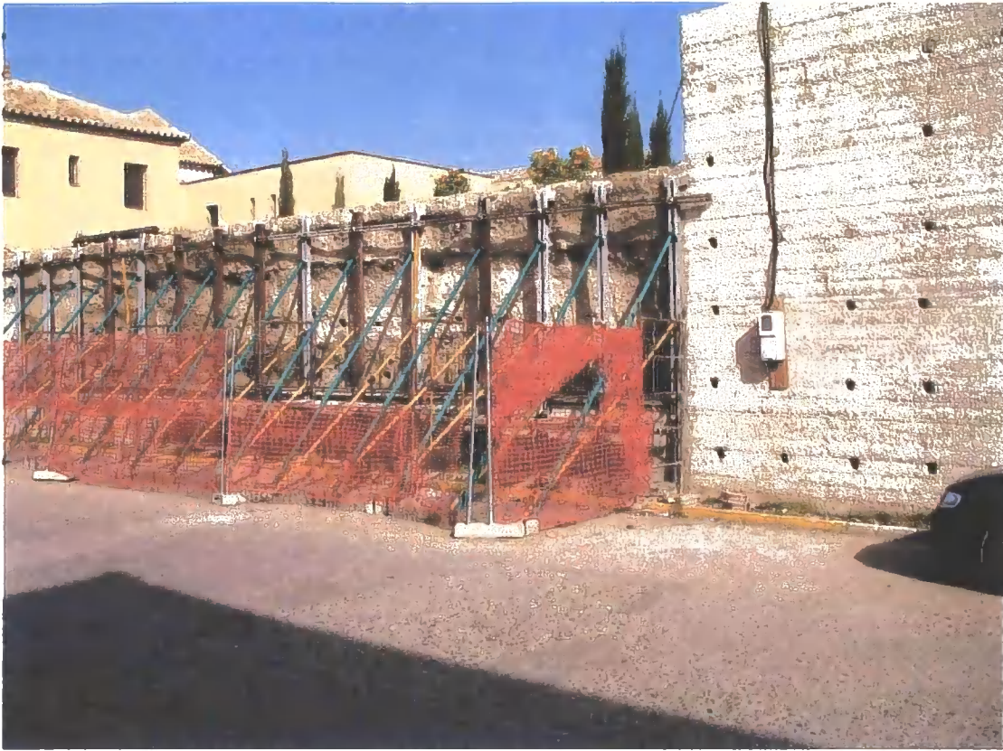
Figure C.78 Pa3 Concrete facing repair to eroded rammed earth wall.
