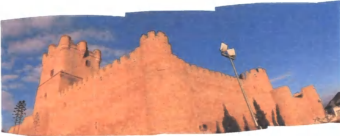
Figure C.93 Vila Villena castle exterior
