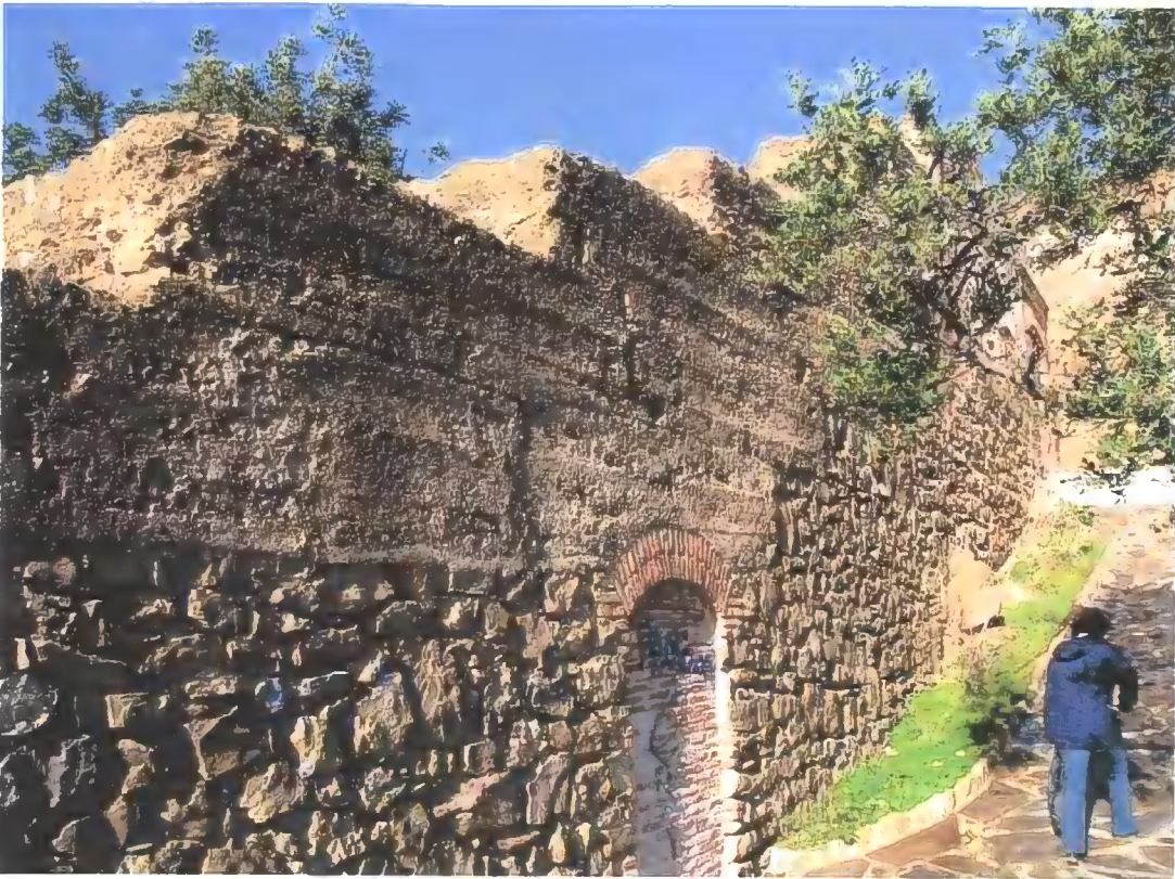
Figure C.68 Ma1 Rammed earth wall above masonry base
