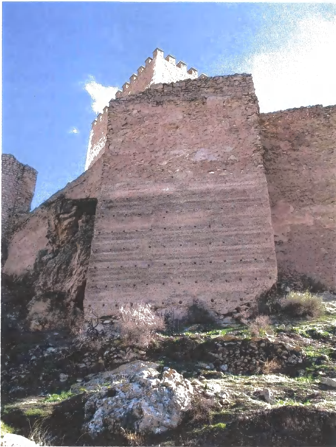
Figure C.67 Lo1 Rammed earth tower base at west end of Lorca castle
