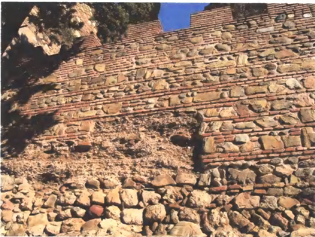
Figure C.69 Ma2 Brick and stone repair to rammed earth wall
