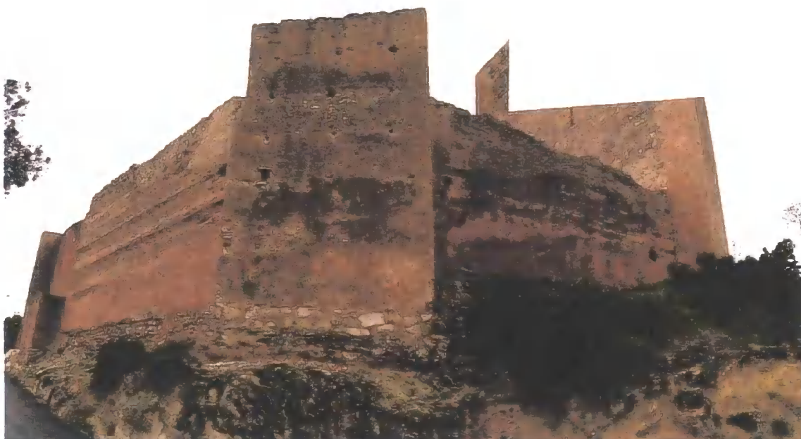
Figure C.71 No1 Rammed earth corner tower
