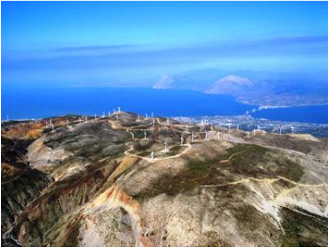
Figure 2-6 Panachaiko Windfarm from SSE direction
