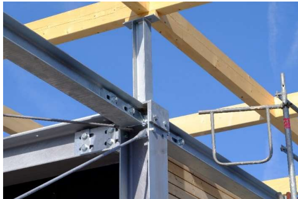
Figure 8 Photo shows complex joints where members meet in multiple directions
