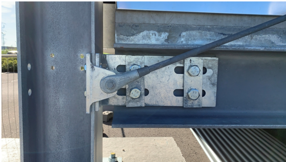
Figure 5 Photo displays the proposed standard distance between the centreline of a column and the end of a beam 1422x800mm (72 x 72 DPI)
