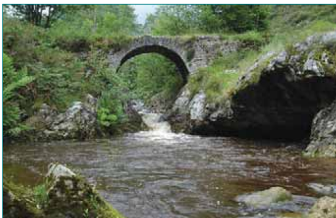
Bridge footings well above trashline height.
