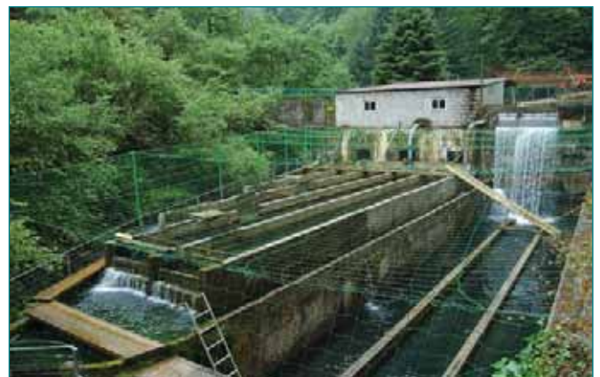
Dilapidated fish farm on the Río Purón; upstream from Picos-18.
