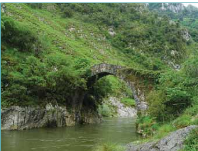
Roman stone-arch bridge on the Río Cares, near Trescares.
