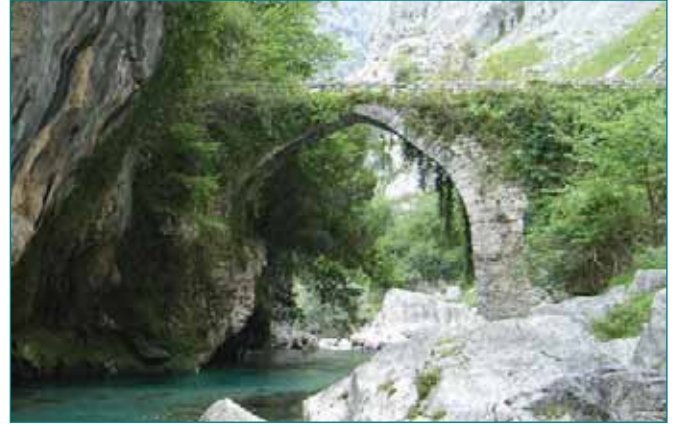
Bridge reinforcement for historic bridge supports high up the bank make no impact on the channel; Picos-19.
