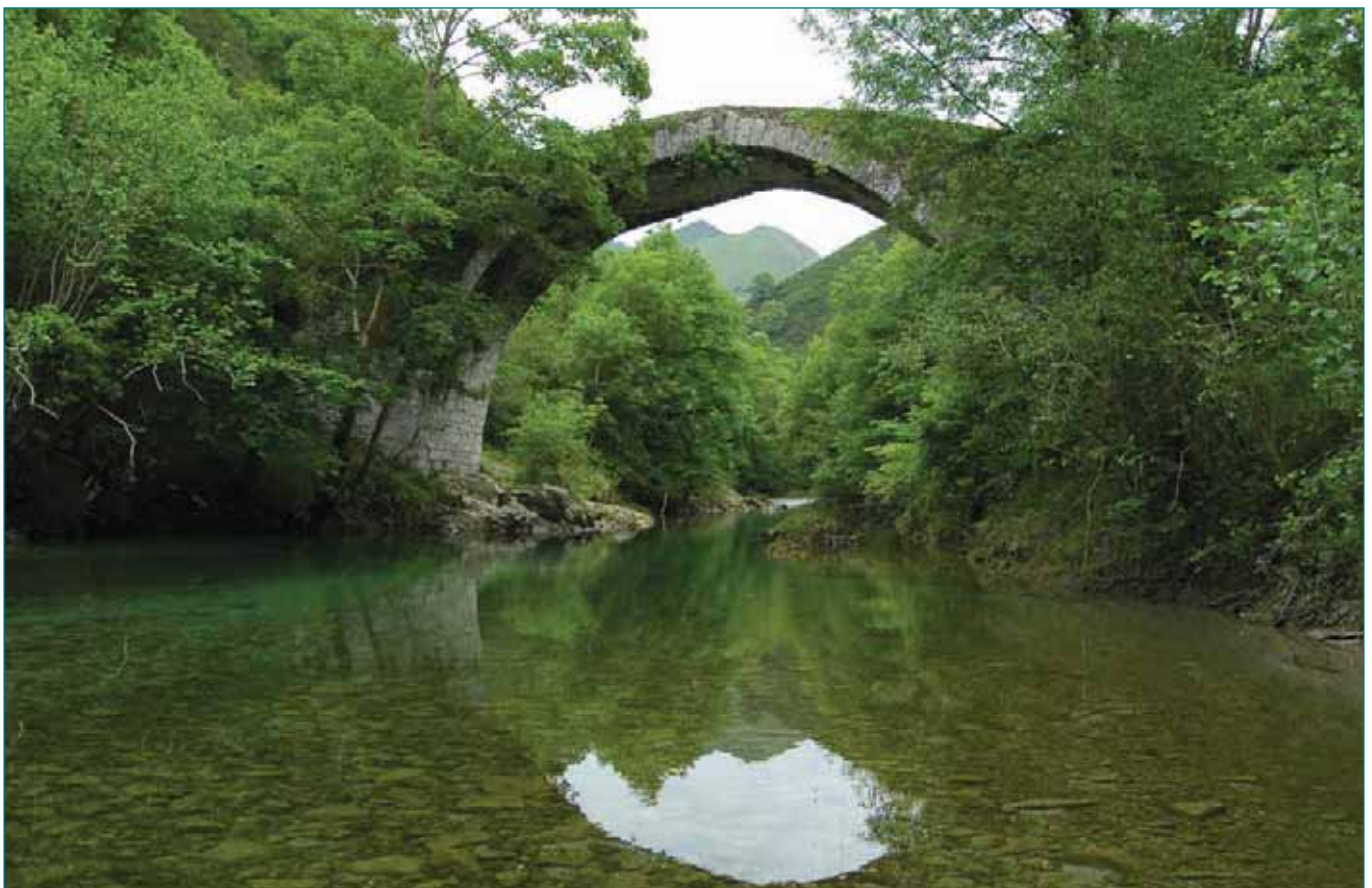
Roman bridge; Rio Dobra, downstream from Picos-12.
