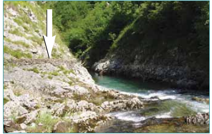
Encased water pipe (arrowed) above trashline level; Río Dobra; Picos-10.
