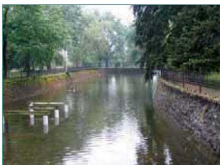
Artificial reprofiling and reinforcement of the banks and channel produce a high HMS score.
