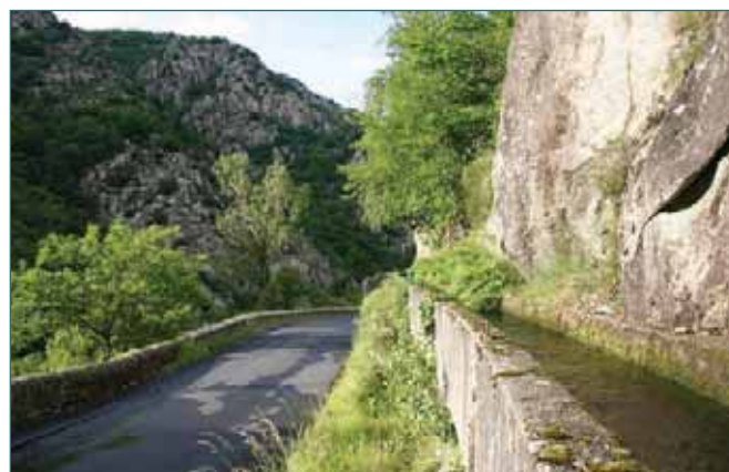
Channels diverting water within a catchment complicate hydromorphological assessment; SE France.
