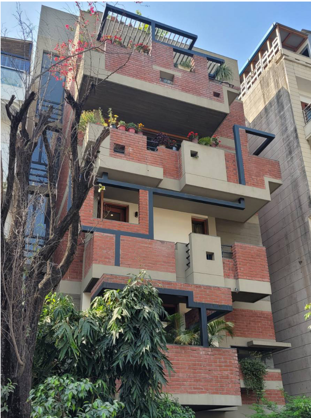
Figure 2: (a) (above) The actual building and (b) (overleaf) an early-stage sketch plan.
