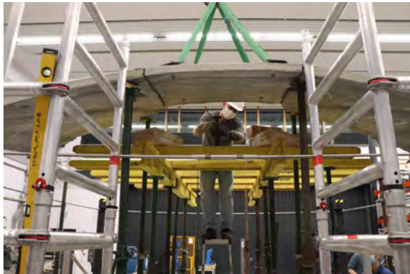
(c) Completion of first arch ©Mishael Nuh
