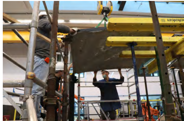
(b) Positioning of corner segment ©Pieter Desnerck
