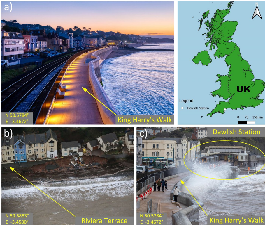
Fig. 1 Location of Dawlish railway station. a The completed section of the new seawall looking towards the train station along King Harry's Walk (Completed first section of Dawlish seawall at dusk (networkrailmediacentre.co.uk)). b An aerial view of the seawall damage sustained at Riviera Terrace in February 2014 (Dawlish aerial view of 2014 damage (networkrailmediacentre.co.uk)). c Waves impacting the newly constructed seawall south of the station, now 2.5 m taller with an integrated wave return (The completed first section of new seawall effectively deflecting waves back out to sea (networkrailmediacentre.co.uk))
