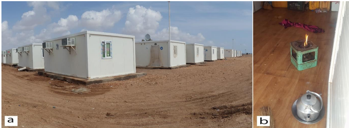
Figure 10: (a): Prefabricated shelters in Markazi refugee camp, Djibouti; (b): Kerosene stove. Photos credits: authors
