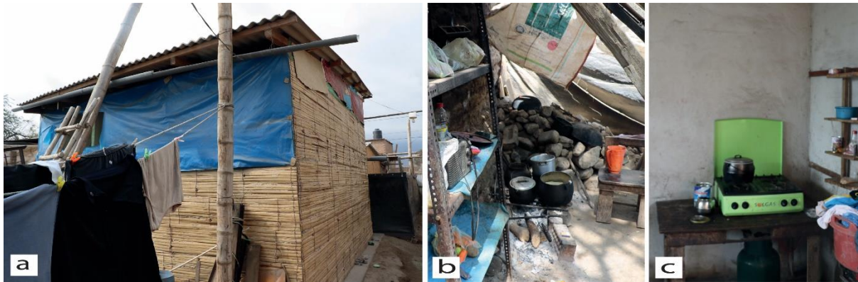
Figure 7: Viru, (a): shelter type 1: high level openings covered with tarpaulin to protect from the cold. (b) external cooking using wood fire; (c): internal cooking using a gas hob. Photos credits: authors
