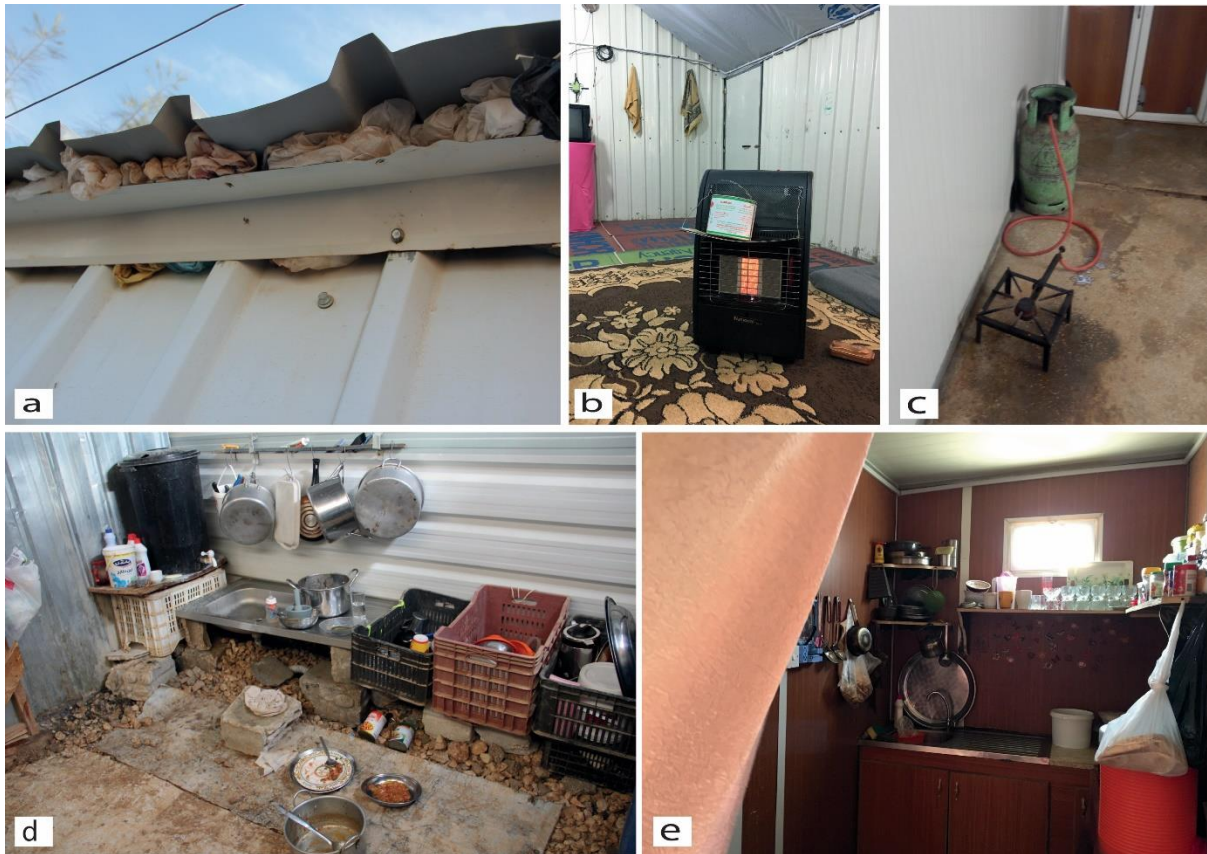
Figure 3: Azraq & Zaatari refugee camps. (a): plastic bags used to fill in gaps in the structure to prevent sand ingress; (b): gas heater used in winter; (c): examples of gas cookers used inside shelters; (d): example of makeshift external kitchen; (e): example of an internal kitchen separated from the living and sleeping space with a curtain. Photos credits: authors.
