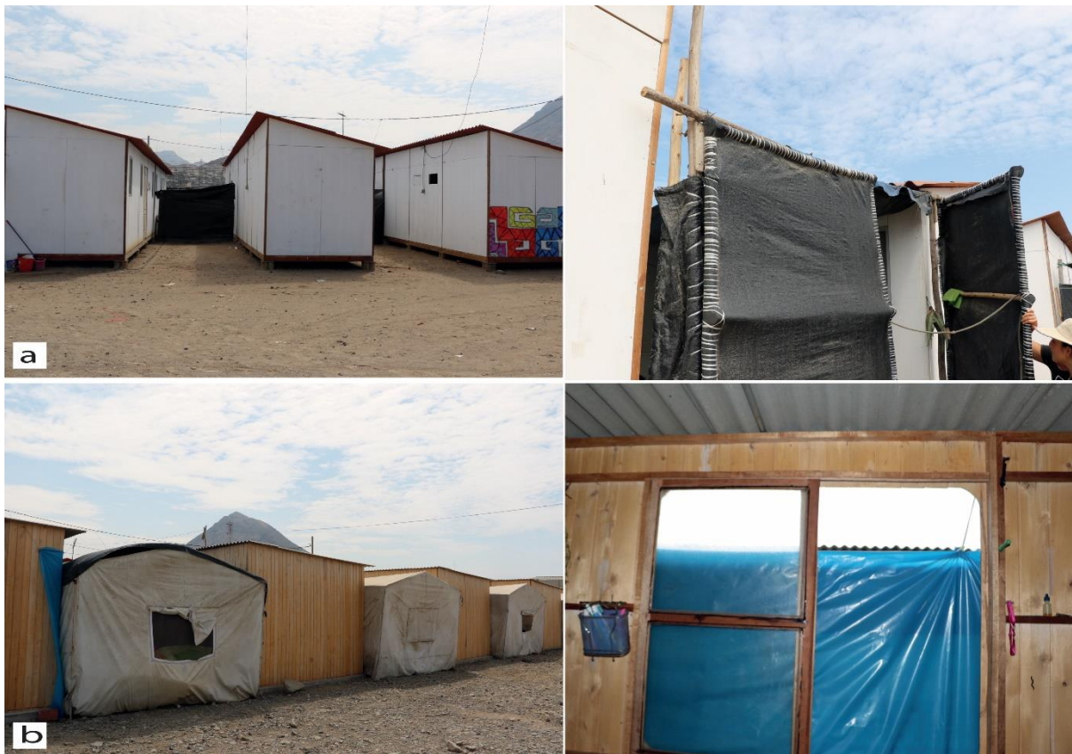
Figure 6: La-Esperanza camp, makeshift extensions between shelters restrict ventilation, (a): shelter type 1; (b): shelter type 2. Photo credits: authors
