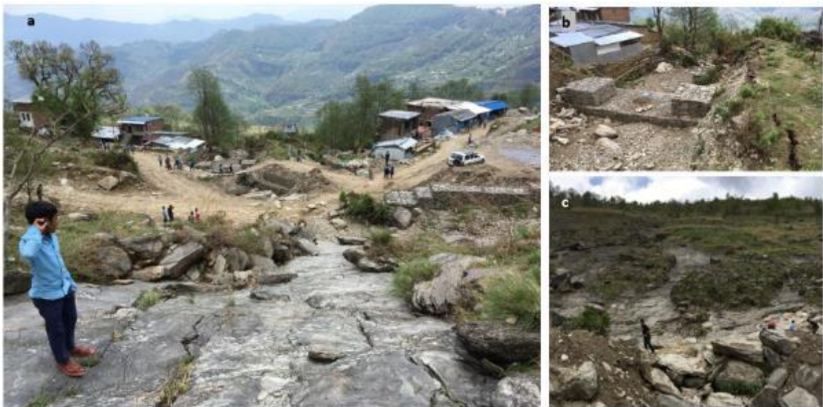
Figure 8. The community of Phulkarka is at risk from high stream flow, overland flow and landsliding. (A) The slopes above the community are widely stripped of their soil cover and this results in very rapid and destructive floods during the monsoon. A system of gabions is being constructed to direct flows and reduce their erosion potential. (B) A close-up of a gabion structure intended to control flow in a stream channel. Bank stability is still very poor (large cracks are visible) and housing is in very close proximity to the stream channel. (C) an view of the slopes above the community highlights the absence of suitable slope and vegetation cover. It is reported that the treeline visible to the left were planted by the community in an attempt to stabilise a landslide.
