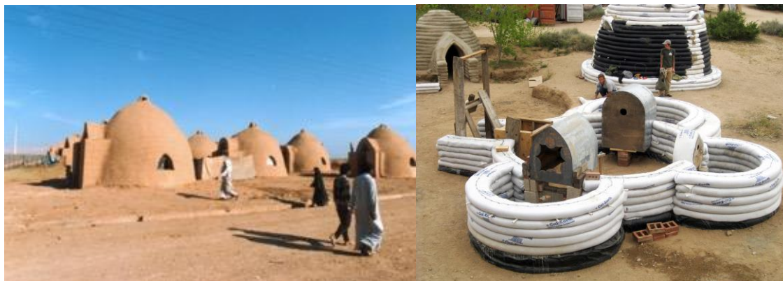
Figure 3: Left: Baninajar Refugee Camp in Iran, 1995; Right: Superadobe construction technique, (Photo credit: Calearth.org, 2017)
