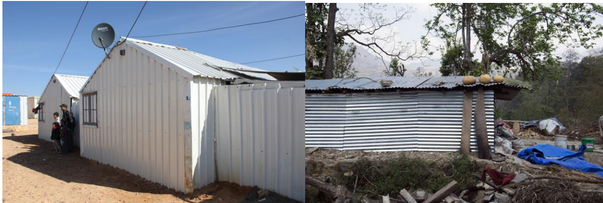
Figure 4: Shelters made of metal sheeting; right: Nepal (photo credit: Emil Helotie, IFRC); Left: Azraq camp, Jordan (photo credit: S.Coley)
