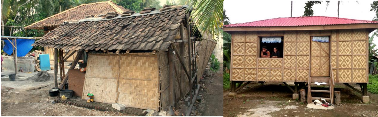
Figure 5: Bamboo and timber constructions; right: Philippine (photo credit: Jenelle Eli, IFRC); left: Indonesia (photo credit: IFRC)
