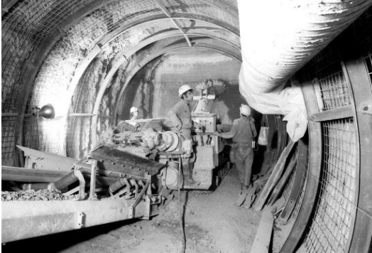
Figure 2. Excavation of TT10 tunnel.
