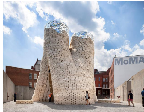
FIGURE 1. Mycelium Brick Tower Hy-Fi On MoMA, By The Architectural Team The Living 2014
