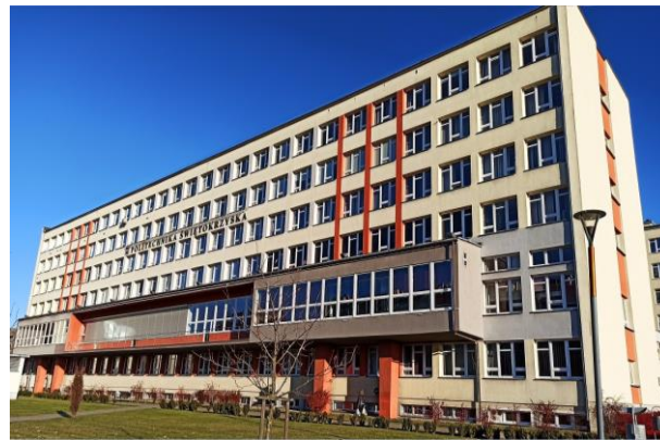
Figure 2. Traditional building “A”—Western façade.
