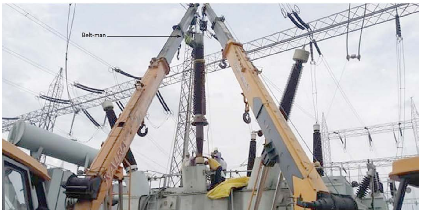
Figure 6. Lowering a 420 kV bushing by means of two Hydra long-boom cranes
