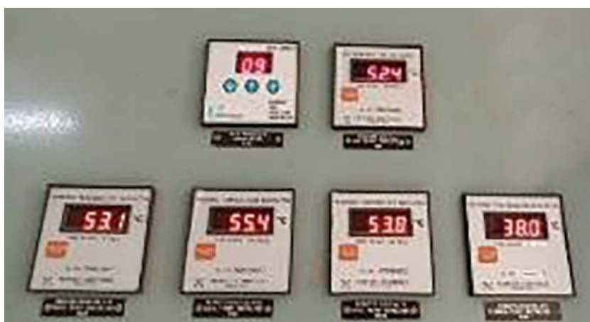
Figure 12E. Remote display meters of WTI and OTI on RTCC pane
