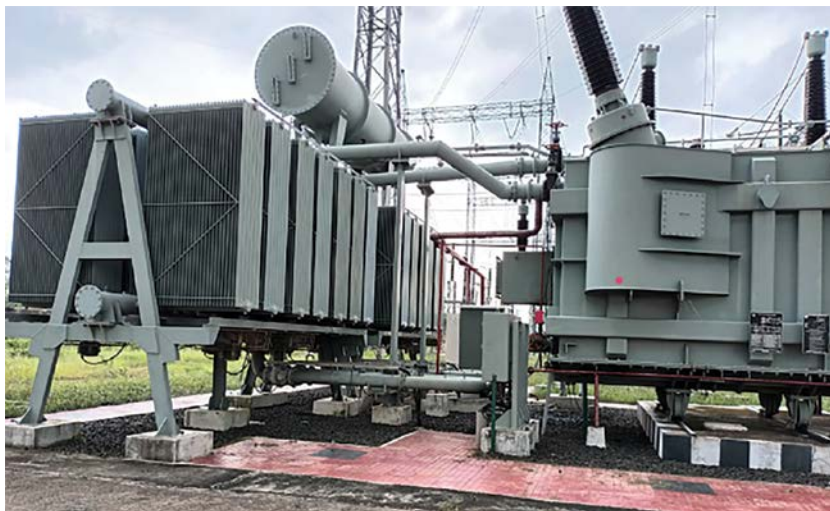
Figure 13B. Externally mounted radiators
