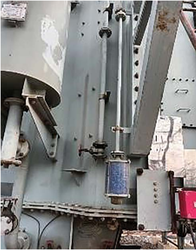
Figure 11A. Silica gel breather
