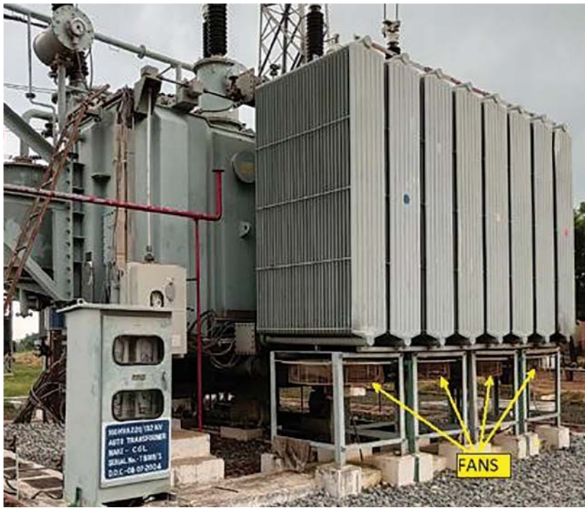
Figure 13A. Body mounted radiators
