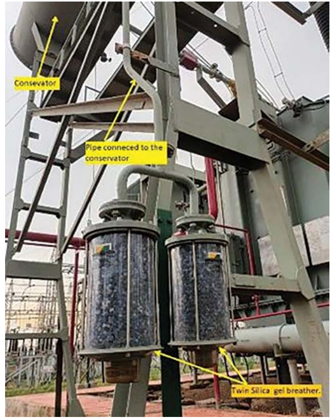
Figure 11B. Twin-silica gel breather in service
