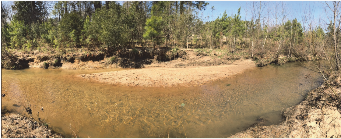
Figure 1. Severe streambank erosion in a restored sand-bed stream in North Carolina. As a result of channel widening due to streambank erosion, the stream's sediment transport capacity has been reduced, causing bed material deposition along the bank. Flow is from right to left.
