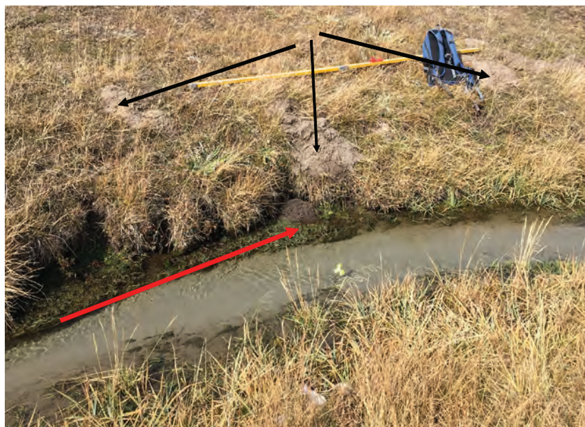
Figure 10. Photograph showing how fine sediment, potentially mobilized from rodent burrows or weakened streambanks (black arrows), has moved into Littlefield Creek and accumulated on the streambed (red arrow) or moved downstream. Photograph by Cheryl A. Eddy-Miller, U.S. Geological Survey, 2018.
