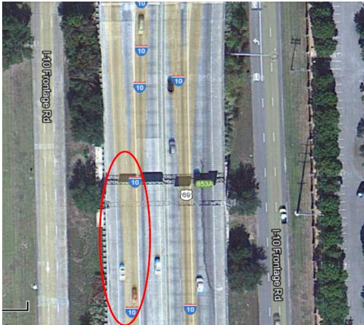
I-10 in Beaumont, Texas - Distressed Portion of the Roadway
