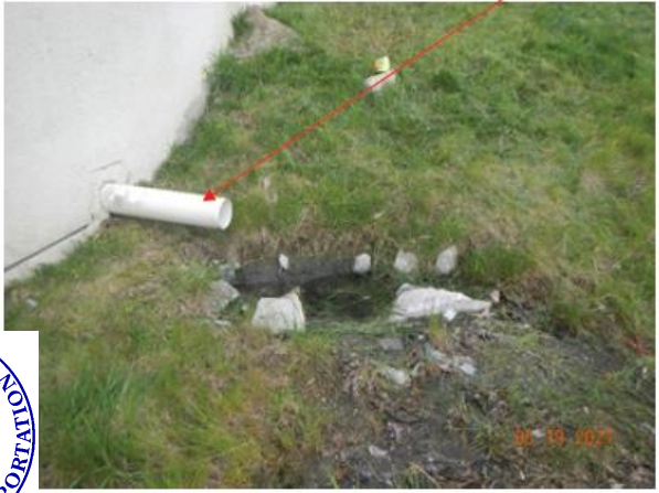
Abutment 1: Northwest Corner
