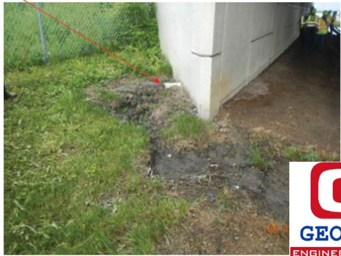
Abutment 1: Southwest Corner
