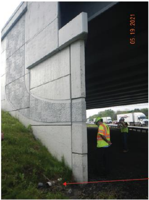
Abutment 3: Northeast Corner
