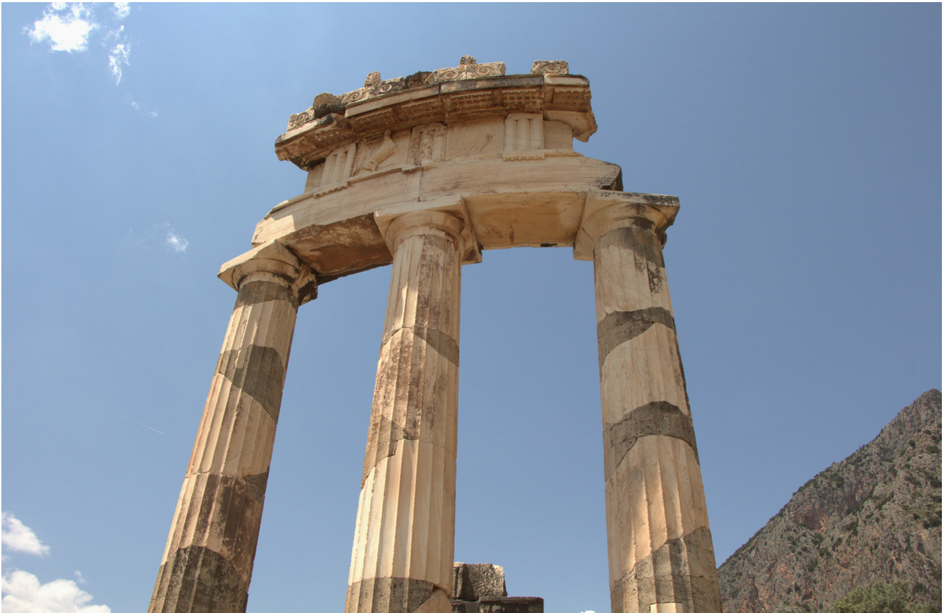
FIGURE 2. Close-up detail of the temple’s partial physical reconstruction. The lighter colored stone in the image is new marble used to fill in missing segments of the temple. Photo taken by author at the Marmaria site in Delphi, Greece, May 2022.
