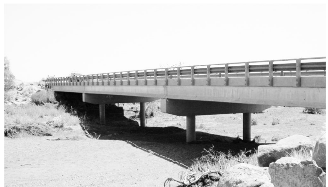
Figure 1. General view of bridge No. 852
