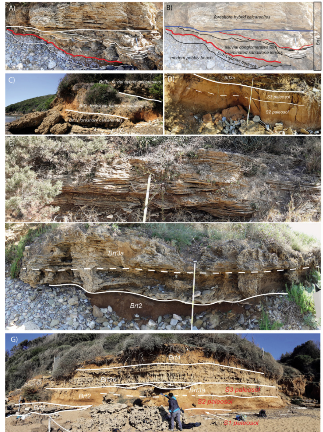
Fig. 23 - A) Outcrop 1a: detailed view of the unconformable contact of unit Brt1 on the deeply weathered subligurian bedrock, hammer for scale; B) interpretative line-drawing of A; outcrop 1b: C) the stratigraphic relation among units Brt1, Brt2 and sub-unit Brt3a; D) particular of the Brt2 deposits with S1-S2 palaeosols, rod is 1 metre for scale; E) detail of the trough-cross laminated calcarenites of sub-unit Brt3a visible few metres southward from C, rod is 0.6 metres long; F) the deeply erosive contact of sub-unit Brt3a on unit Brt2 few metres southward E attesting to an high relief erosional contact between these deposits, rod is 1 metre long; G) outcrop 1c: panoramic view of the succession at this outcrop annotated for the stratigraphic features described in the text, person for scale.
