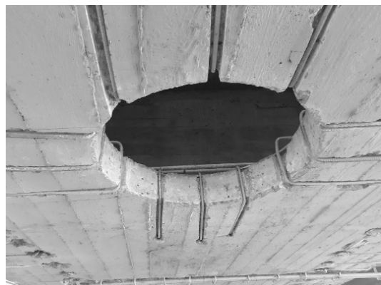
Figure 20. New openings in the counter-slab/ Nuove aperture in controsoletta.
