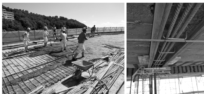
Figure 18. Reinforcements in the slab and crossbeams/ Rinforzi in soletta e traversi.
