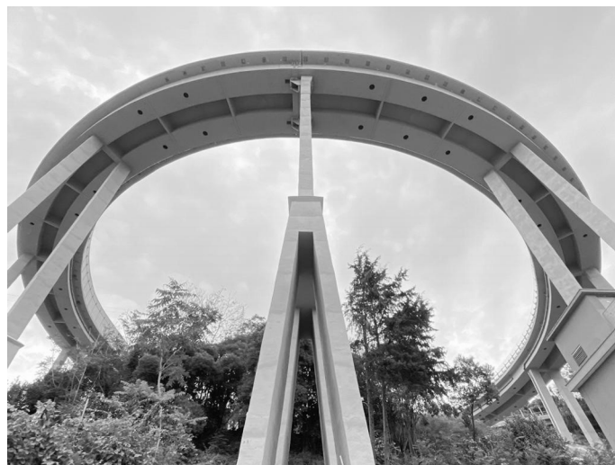
Figure 24. The helical ramp at the end of the works (2020) / La rampa elicoidale al termine dei lavori (2020).
