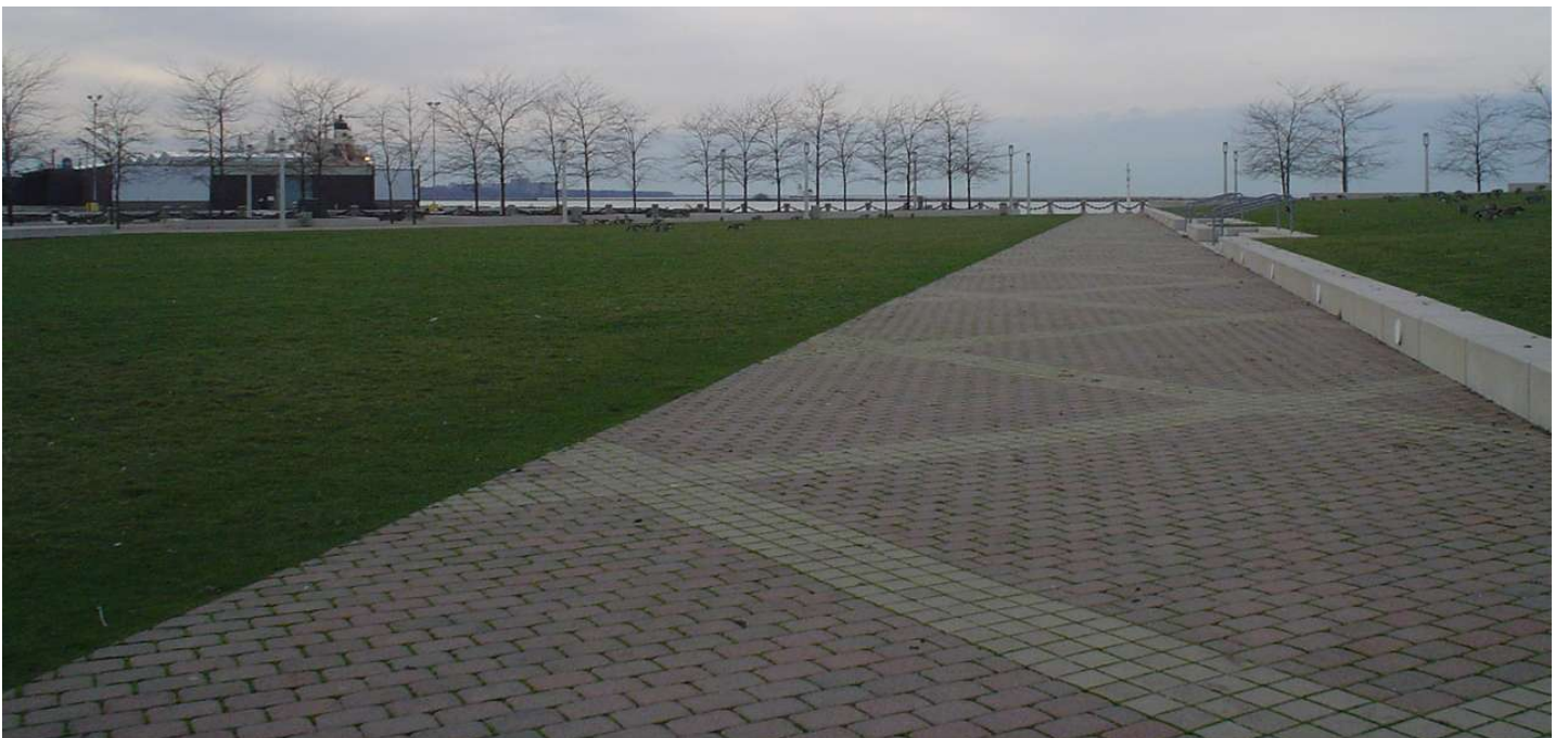
Voinovich memorial park - Looking Northwest
