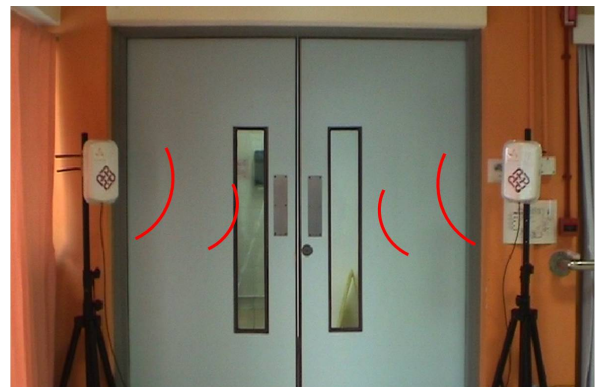
Fig. 4b. RFID Gateway in each room
