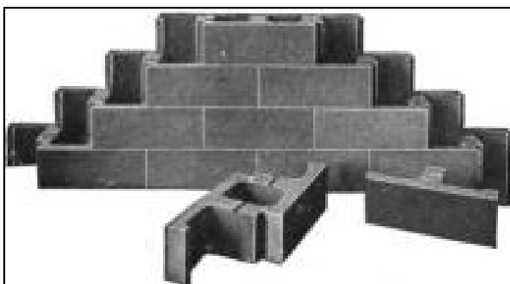
Figure 13: An example of a two-piece wall system. Two-piece wall block was typically built by mechanical concrete block machines. This block design was manufactured by the American Hydraulic Stone Co., Rice, 37.
