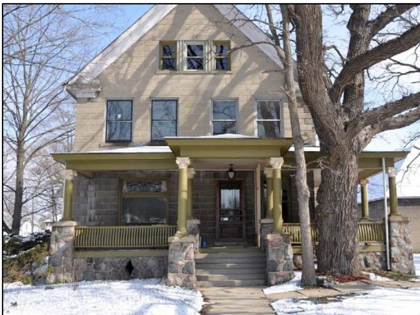
Figure 15: Concrete block home built with an American Hydraulic Stone Co. machine, c. 1905-1906. The home was built with panel-face block. Marengo, IL. Photo taken by James Hall.
