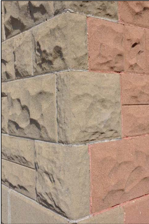
Figure 18: An example of red concrete block. Red concrete block was manufactured by mixing oxide of iron with the cement. This mixing was done prior to the cement being mixed with aggregates and water. Photo by James Hall.
