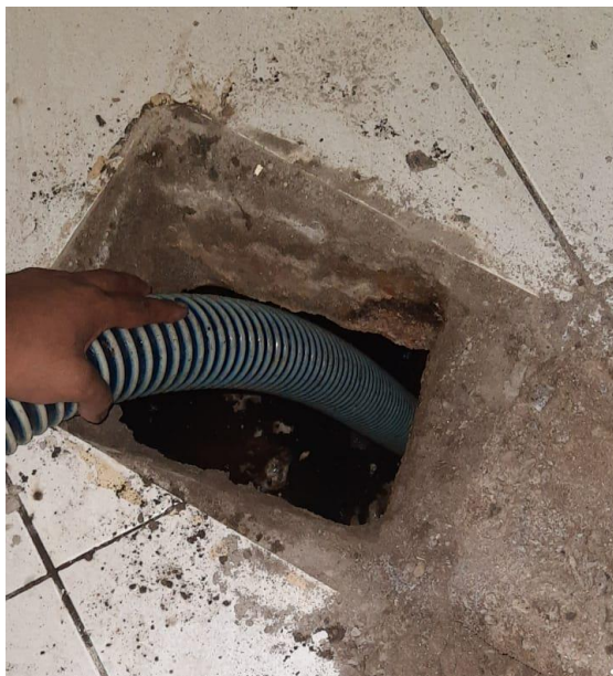
Figure 5. Fecal sludge suction process from septic tank
