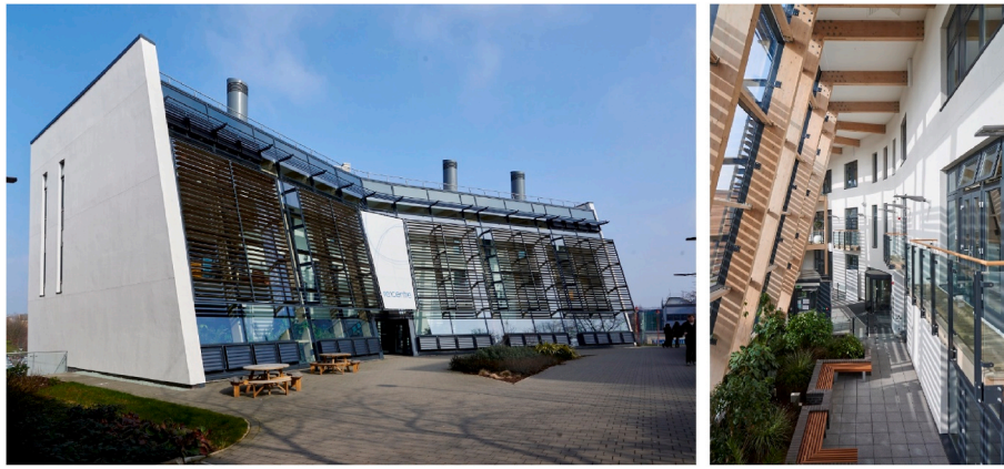
Fig. 5. Bright Building, the world's largest monolithic hempcrete building (Image courtesy: Future Constructor & Architect).
