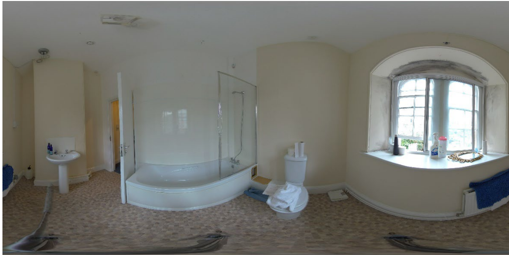
Figure 3. A 360 photosphere of the internal of the upstairs bathroom of the house used for simulation walkthrough housing inspection. (Note the simulated damp and mould hazard around the window frame.)
