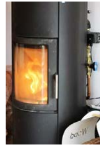
(f) Hydronic stove in Norway.
