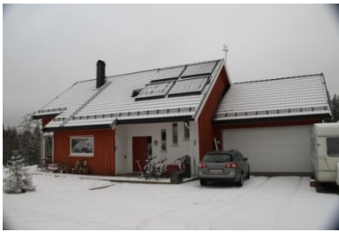
(a) Hydronic stove and solar panels in low energy house in Norway
