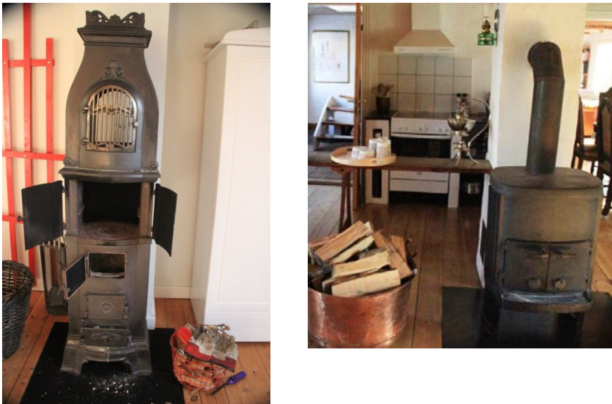
Figure 1-1 Cast-iron stoves found in a rural home in Jutland (Denmark): classical iron stove on the left hand side in a room and cast-iron cookstove 4 in the kitchen on the right hand side.
