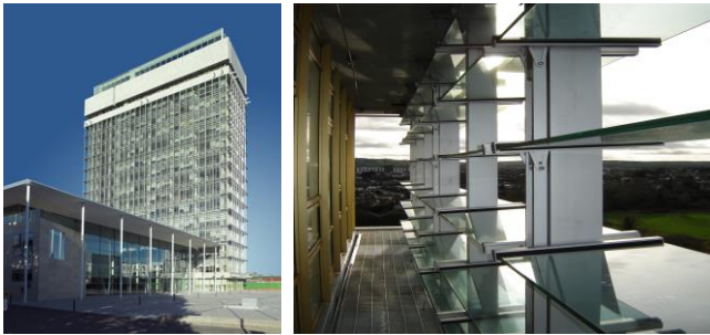
Figure 1: External View of the refurbished building (left) and detail of retrofitted second skin with automated glazed louvers (right)
