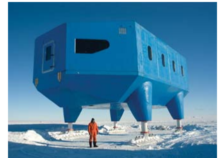
Above: The first completed module of the UK's Halley VI Research Station stands on the Brunt Ice Shelf in Antarctica.
