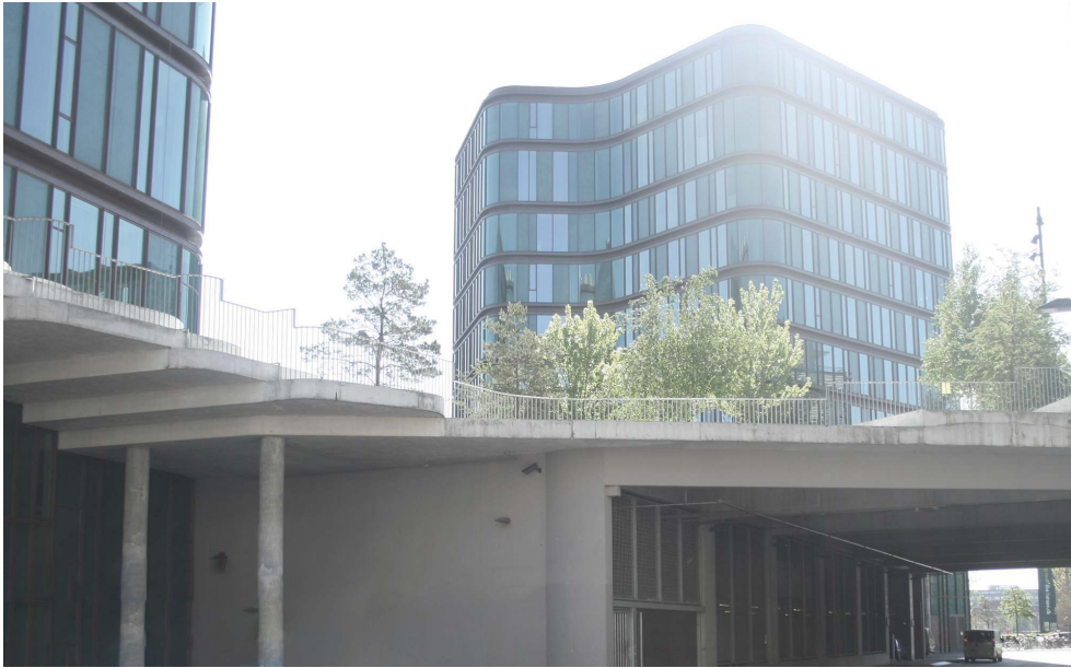
Illustration 5: The parking garage below the green scenery
