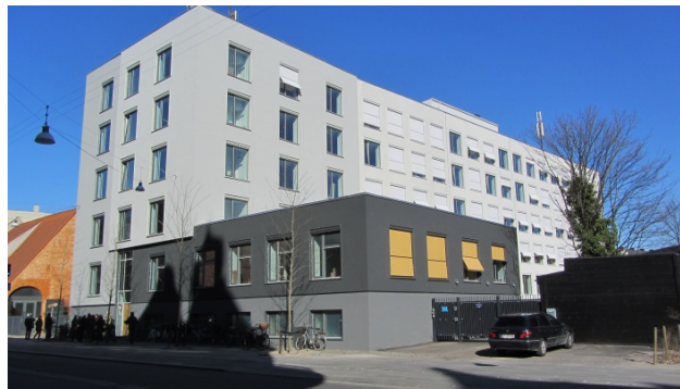
Fig. 3 The office building after retrofit
