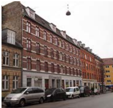
Figure 2. Facade picture of G1. Jernbanevej before renovation and as of today.
