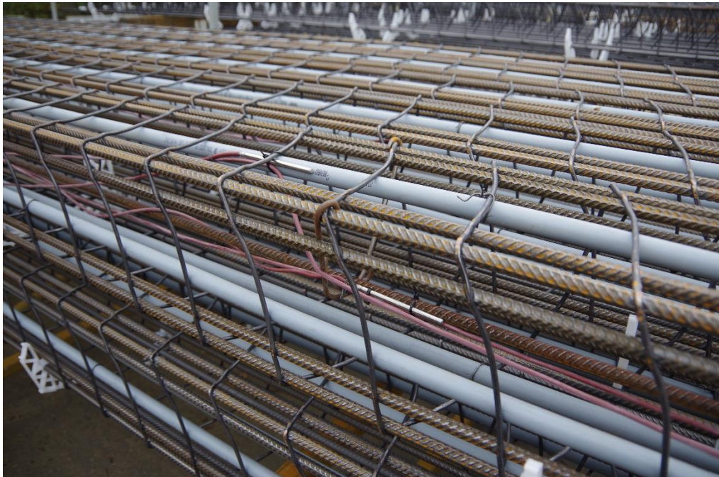
Figure 19: Pile instrumentation with Pt100 temperature sensors.
