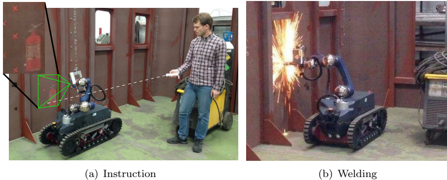
Fig. 6.2: Instruction of welding operations using an IMU pointing device and projection mapping. Welding positions are shown as red crosses and obstacles such as the fire extinguisher can also be shown. Stud positions can be added, deleted, and moved using a cursor controlled by the pointing device.
