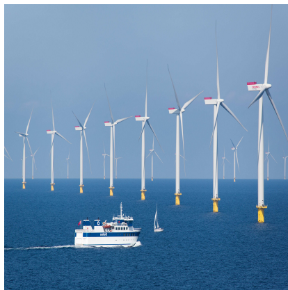
Figure 1.6: Offshore wind farm at Anholt. (Dong Energy 2015)
