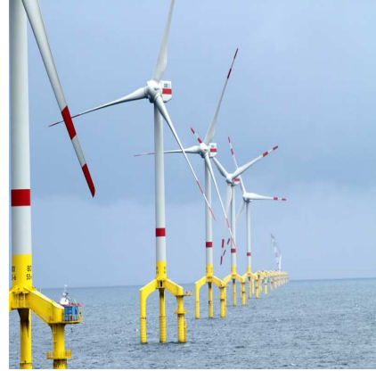
Figure 1.12: Tripiles foundations for the offshore wind farm BARD Offshore 1 in the North Sea. (Bard 2015)
