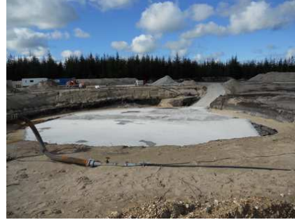
Figure 1.3: Octagonal onshore wind turbine base. (Hamacher 2012)
