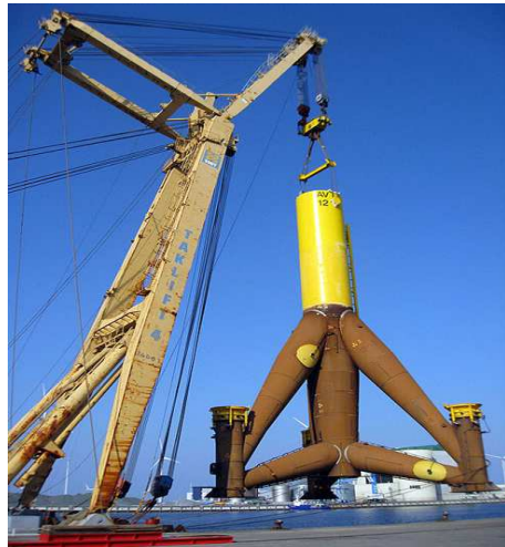
Figure 1.11: Tripod foundations for the ha Ventus offshore wind farm. (Offshore Wind Technology 2015)
