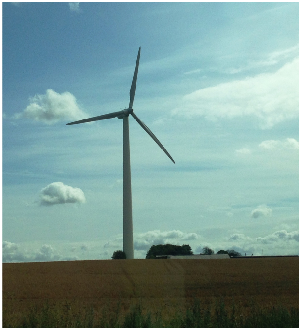
Figure 1.2: Wind Turbine in North Jutland, Denmark near the E45 highway.
