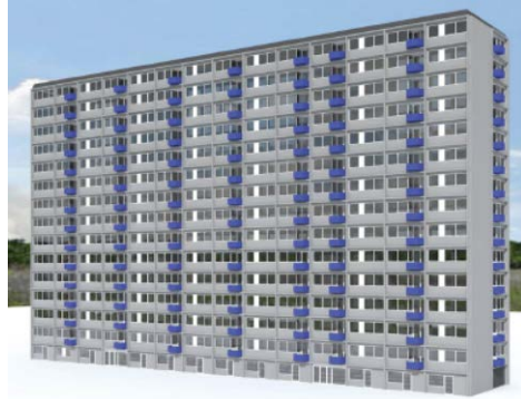
Fig. 2 One of the three Sorgenfrivang blocks prior to refurbishment. Illustration by DOMINIA Consulting Engineers.
