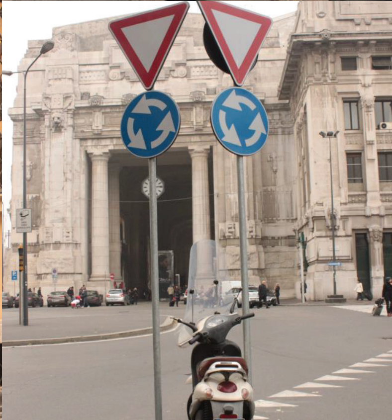
Inappropriate symbol was tempered on the regulatory sign.
