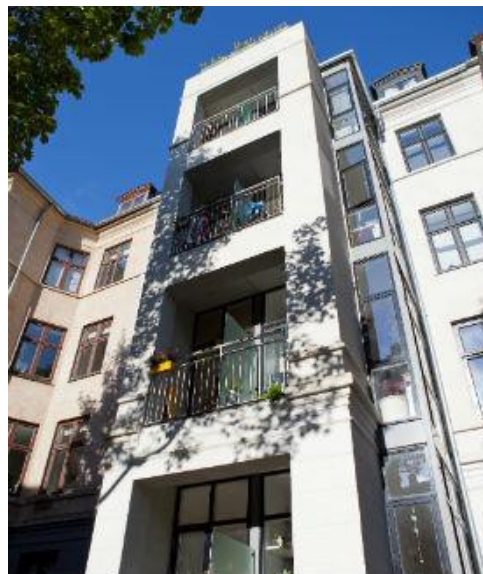
Copenhagen, exterior insulation and new balconies
